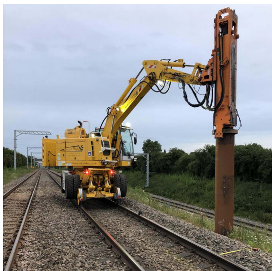
Fig. 13. Pile driving with commercially available plant
