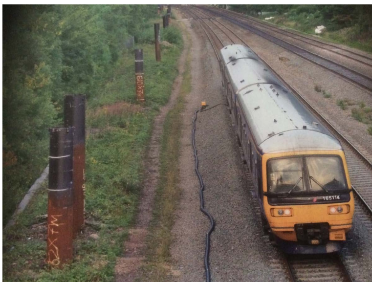
Fig. 12. GWEP - overlong piles which could not be driven offset to avoid signalling cables.
