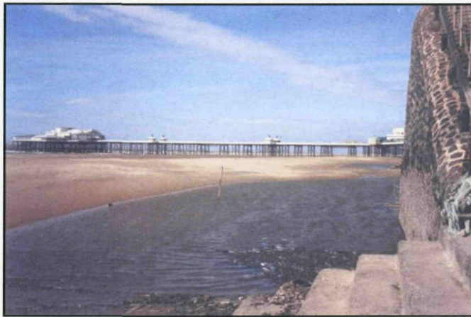
Figure 3-1: Blackpool, UK - A trough at the toe of a vertical seawall (from HR Wallingford, 2005)
