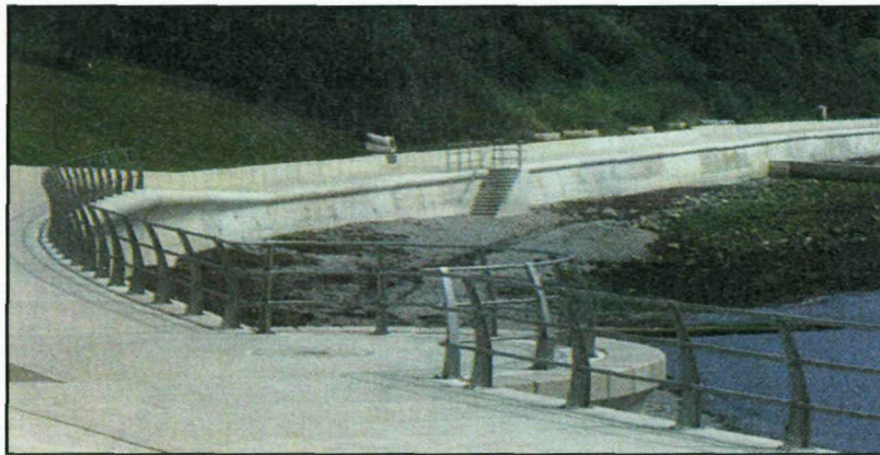
Figure 7-7: Seawall with small recurve, Newton's Cove Coastal protection scheme, Weymouth, completed 2004 (NCE, 2004)
