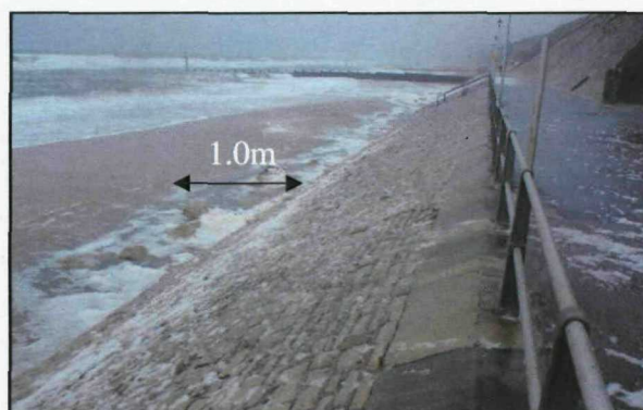
Figure 2-6: Southbourne, Dorset UK. A trough at the toe of a sloping seawall
