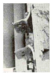
Figure 1.1: WWII Connection damage investigated by Lord Baker in 1948 (Byfield 2006)
