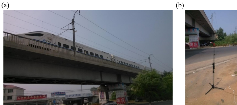
Fig. 11. Images of the vibration and noise measurement: (a) Image of the bridge; (b) Microphone of S2.
