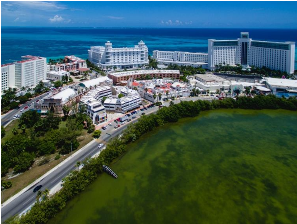
Photograph 3. The construction of many hotels and tourist establishments extend across 23 kilometres (15 miles) along the sea and the lagoon (Santisteban, 2018).
