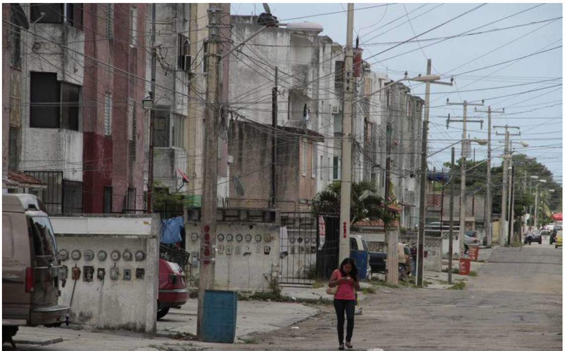
Fig. 27. Roads with buildings without maintenance and in which not all the luminaries work properly making streets not very safe for pedestrians (Nefmex, 2015).
