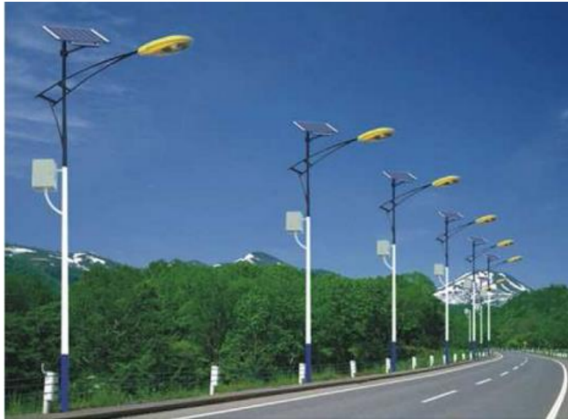
Figure 2.8: Solar-powered streetlights (reproduced from [111]).
