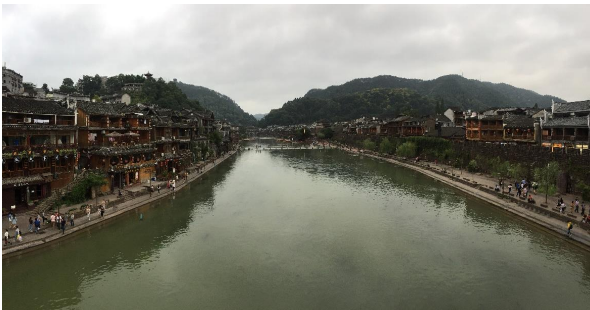
Figure 12 The stilted buildings (Diaojiu buildings 吊脚楼) by the River Tuo 沱江, Fenghuang 凤凰 511
