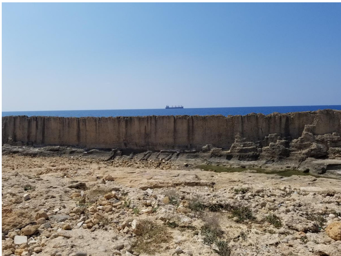
Figure 5.15: The Roman sea wall in Batroun, essentially the result of quarrying activity with an outer barrier left as shelter from wave action (photograph by author)
