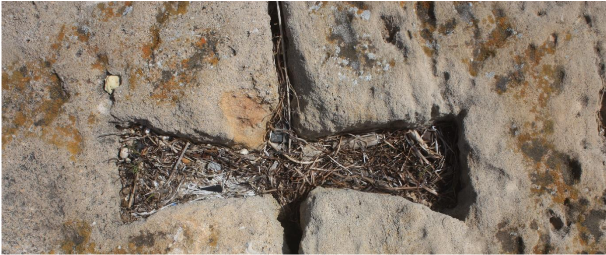
Figure 5.22: Example of dove-tailed joint observed in breakwater at Elaia (photo courtesy of Nicholas Carayon)
