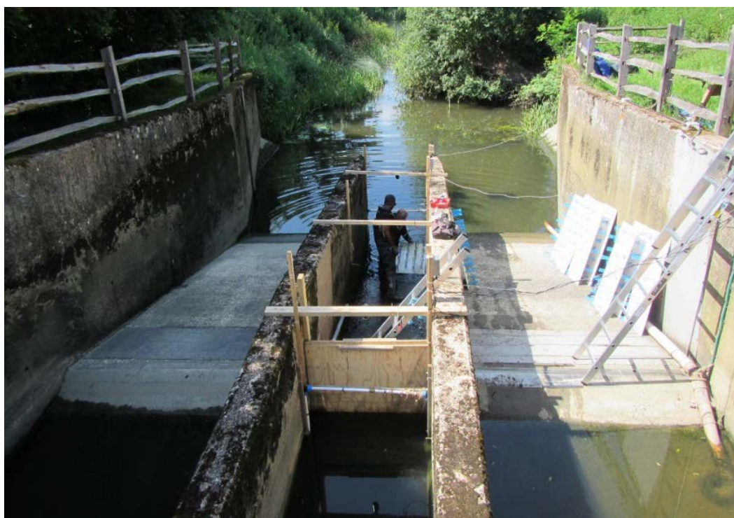
Figure 5.3 Fish pass installation on the compound Crump weir at Sakeham where boards were installed in the central channel and water was prevented from going down the weir during installation using 2 wooden boards held in place upstream.
