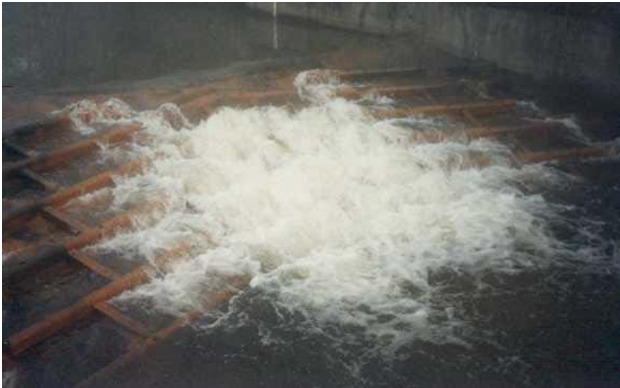
Figure 2.8 Flat-V weir retrofit using low cost baffles on the river Moors at Hurn in Dorset (White and Woods-Ballard, 2003).
