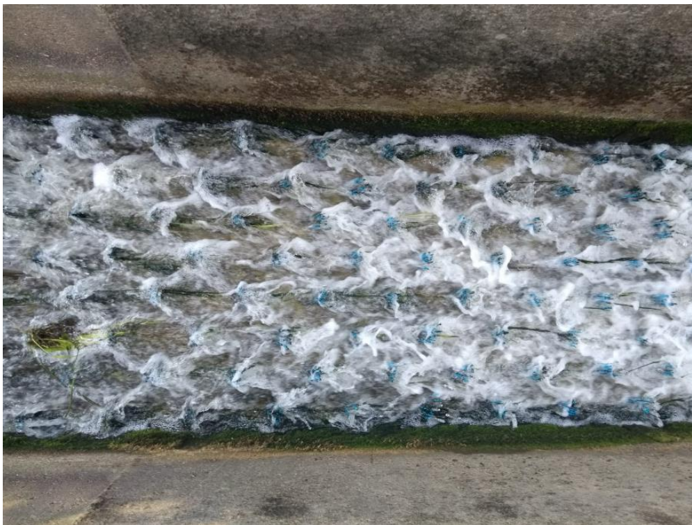
Figure 5.7 Debris accumulation over the fish pass installed on the compound Crump weir at Sakeham in July 2018.
