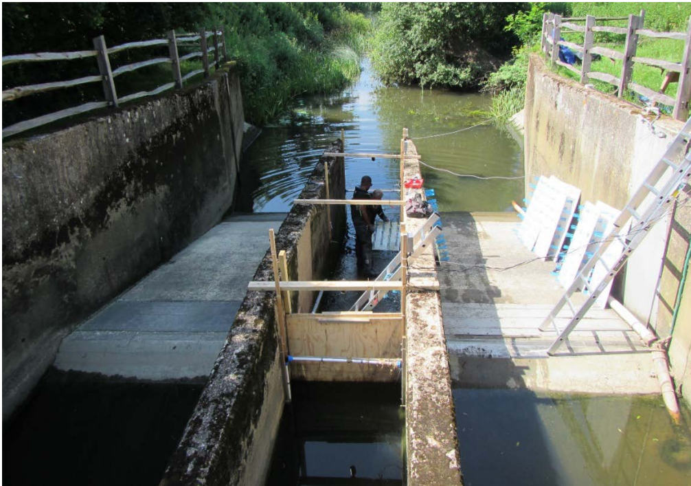
Figure A.3.1 Photograph of the CBCs being installed in the field on a compound Crump weir in the central channel.
