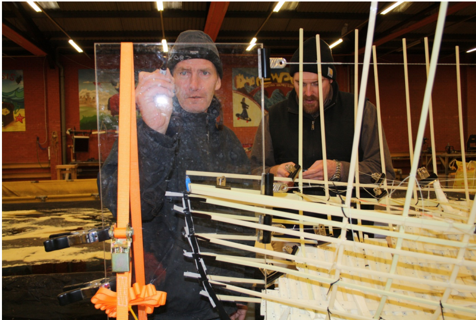
Figure 10-1 Dry-erase markers were used to draw on potential posts and planking termination points during an early iteration of the process. (Newport Museums and Heritage Service)
