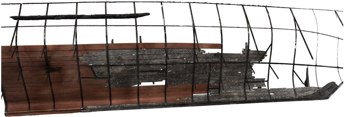
Figure 25 Existing cradle support structure at circa 1m intervals
