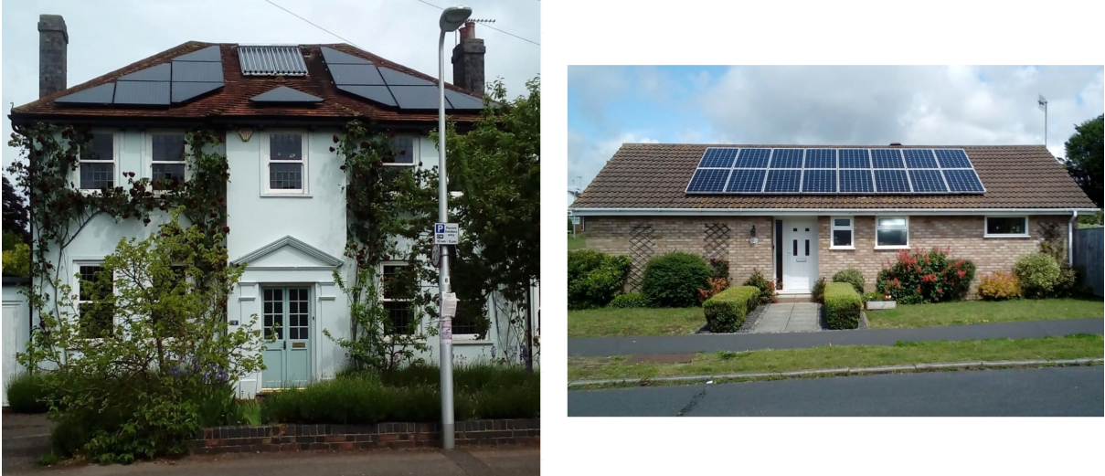
FIGURE 2.14: PV arrays of differing complexity. Left: requiring 9 triangular panels, 4 square panels, and including a solar thermal panel; right: comparatively simple 8 \times 2 array of rectangular panels. Photos by the author.
