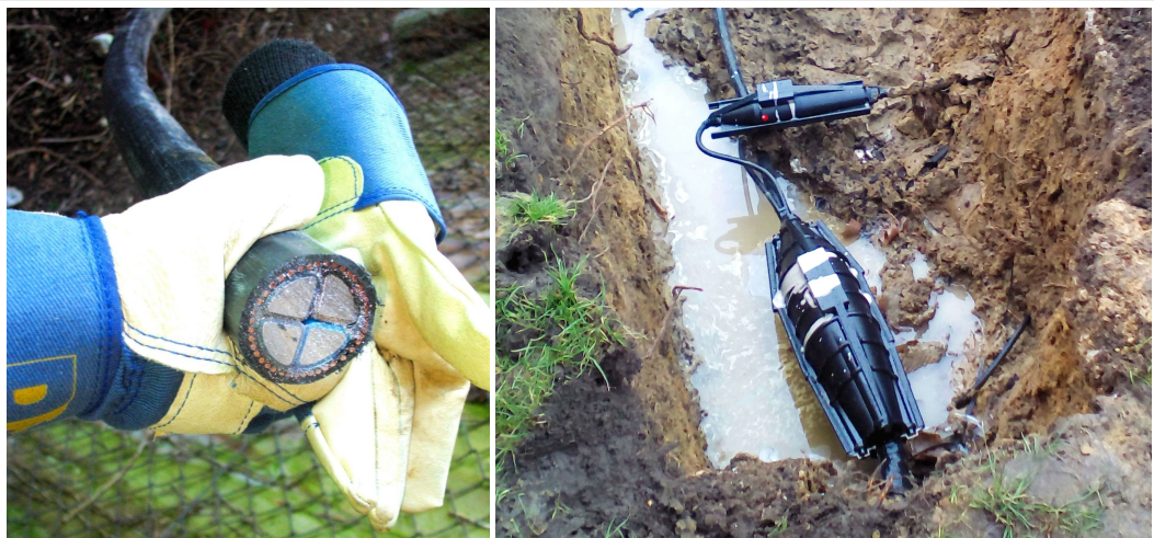
Figure 2-8: Feeder cable (Phases 1, 2, 3, N with Earth outer) and a house take-off
