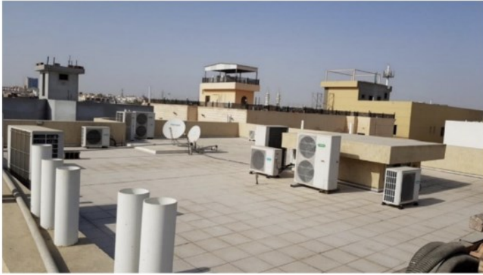
Figure 1. Case study rooftop showing area available for PV mounting of around 200 m 2 which would entail a raised structure to allow space underneath for existing A/C units and plant and to prevent shading.
