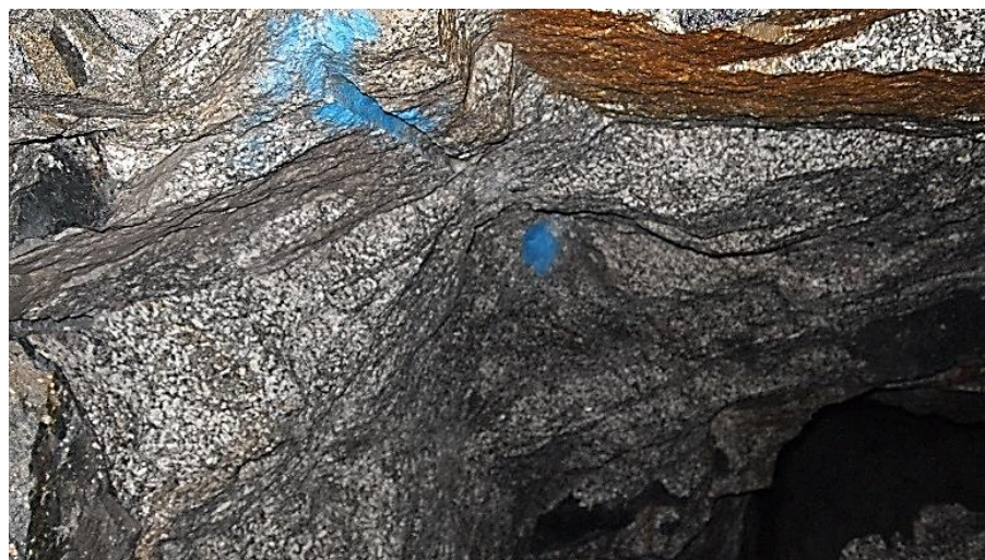
Figure 71 Cross cut expansion post blast detail
