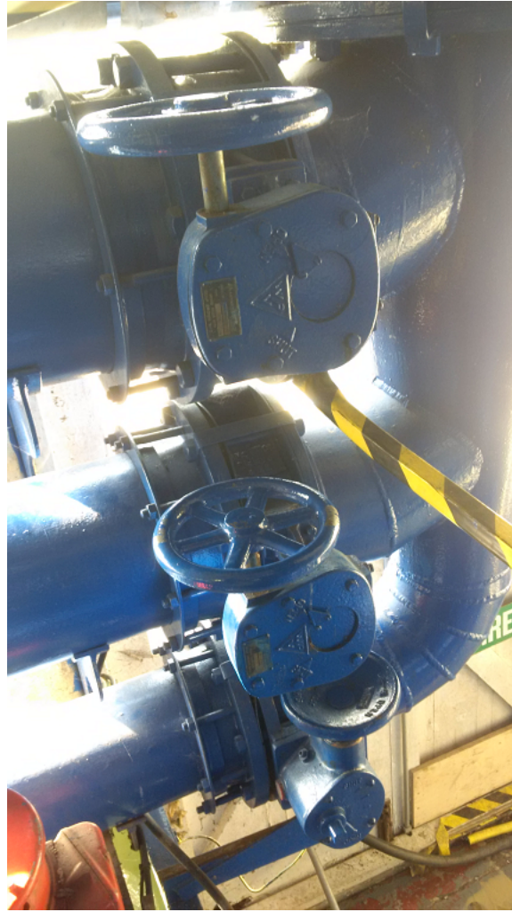
FIGURE 3.3: Regulation valves for the Chilworth Internal flume. Top to bottom: pump 1, pump 3, pump 2.
