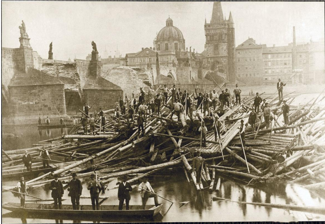
FIGURE D.4: Accumulated debris at Charles' Bridge during the 1890 flood. The photo shows the relatively uniform length logs and the people working on the debris removal. Source: Museum of Prague.
