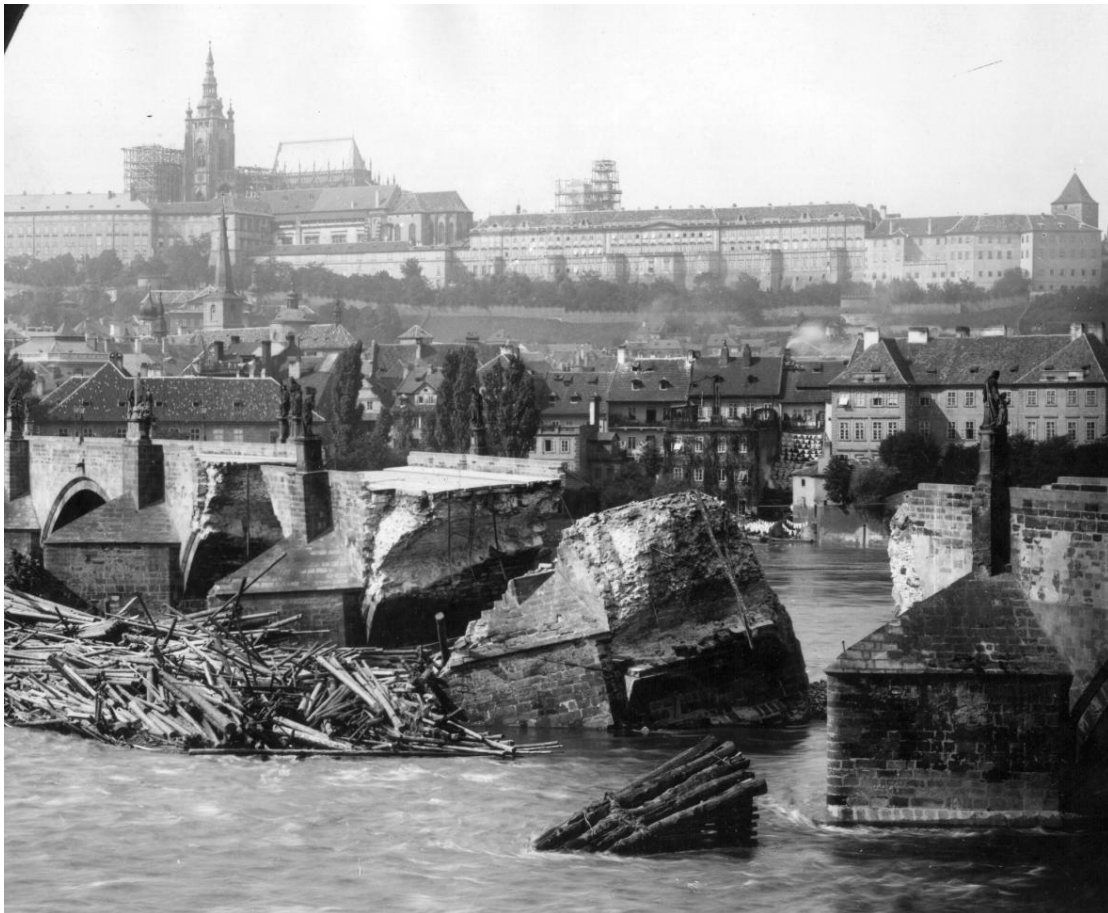
FIGURE 1.1: Charles' Bridge failure occurred during 1890 flooding. Source: Museum of Prague.
