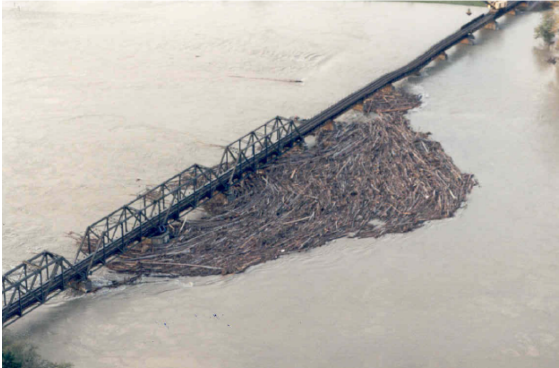
FIGURE 2.6: Large LWD accumulation at the Skagit River, Washington, US, during a flood in 1995. It can be observed how blockage is caused by debris bridging two single-pier accumulations. Source: Washington State Department of Transportation.
