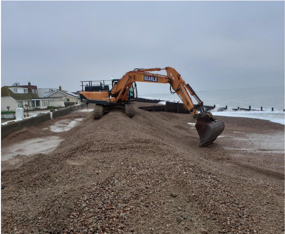
734 Figure 13: Plant is deployed at Hayling Island for emergency repairs to the beach. Photo by Havant Borough 735 Council.
