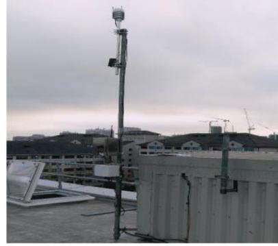
Fig. 1 Weather station at substation of Transformer B.
