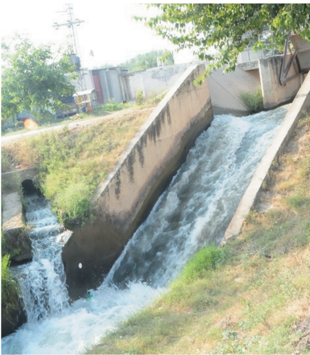
Figure 2. Typical small drop structure (Image: Zia Ul-Haq, with permission).
