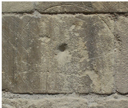
Figure 86 Recorded example of dividers created mark: Chichester Cathedral (authors own image 2014)
