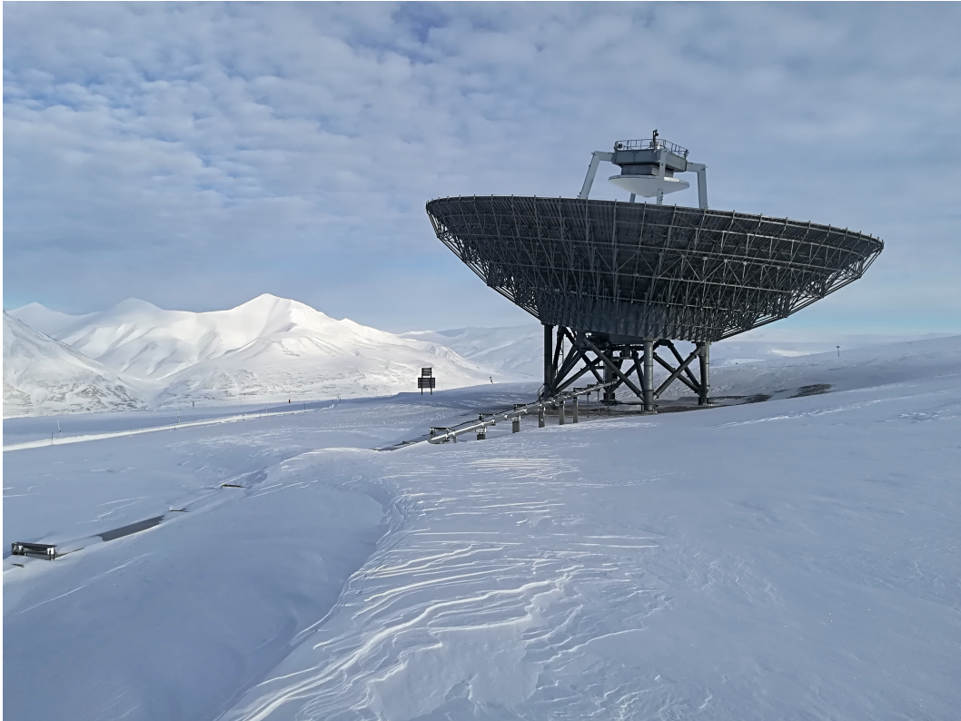
FIGURE 3.4: The EISCAT Svalbard Radar Fixed 42 m Dish. Photo taken by the author.
