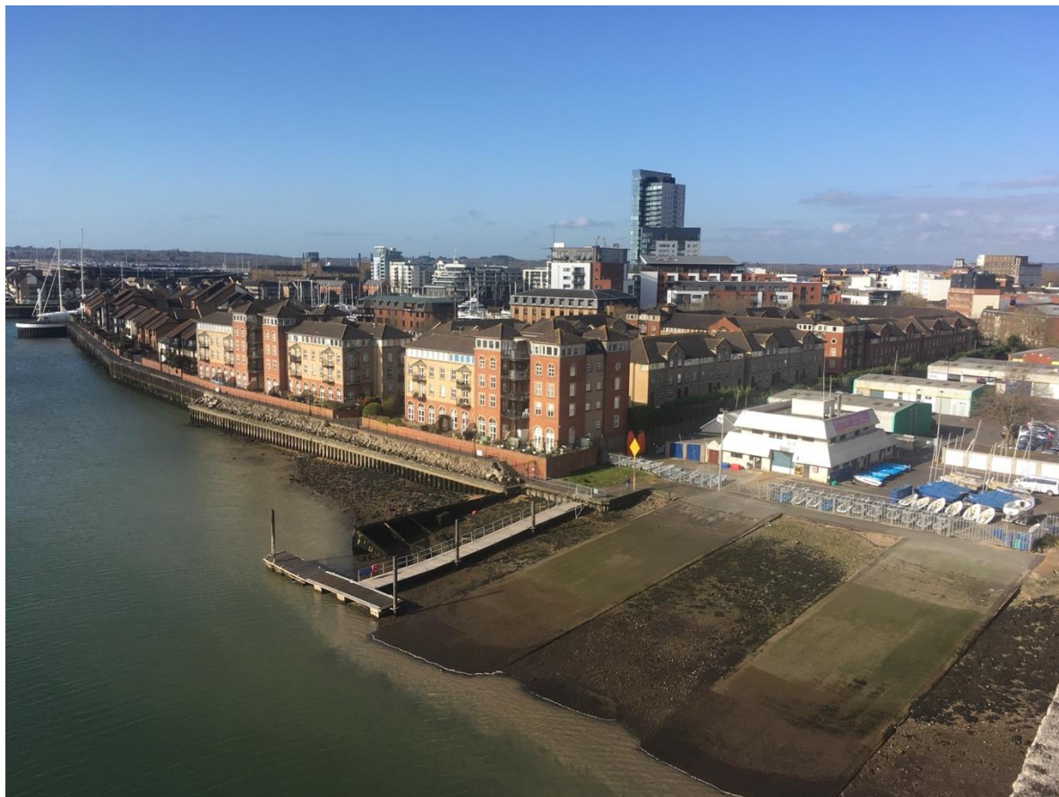
Figure 3-2 Southampton Water Activities Centre at low water (source: author)
