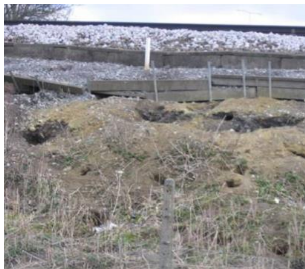
Figure 2-7 Example of burrowing according to NR classification system (Network Rail, 2015a)
