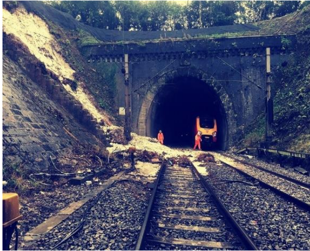
Figure 6-11 Cutting failure at Watford(RAIB, 2017)
