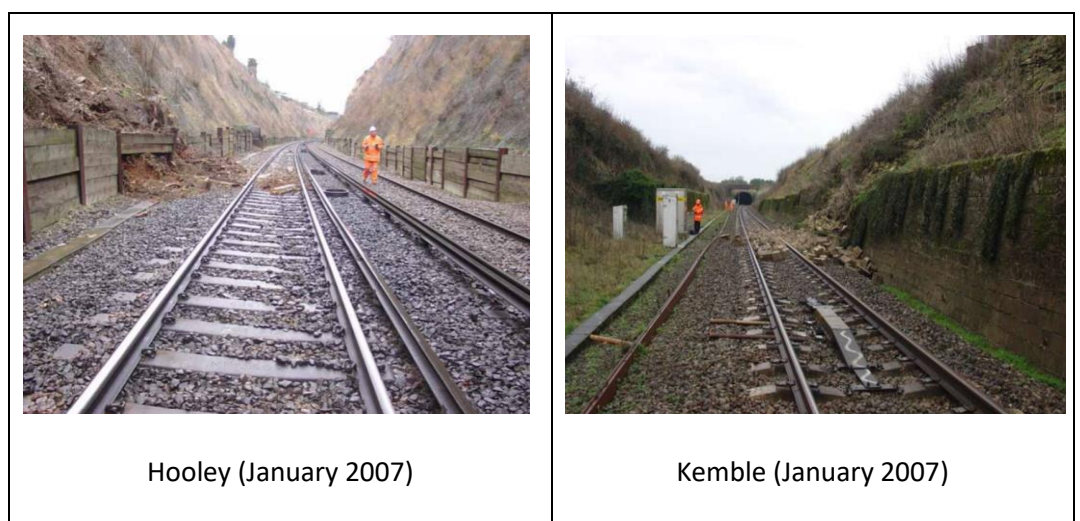
Figure 2-12 Recent cutting failures causing derailments (RAIB, 2008a; RAIB, 2008b; RAIB, 2010; RAIB, 2014; RAIB, 2017;.RAIB, 2018)
