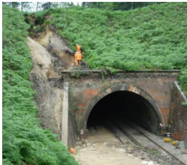
Figure 2-5 Example of washout according to NR classification system (Network Rail, 2015a)
