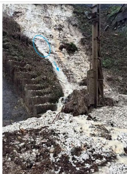
Figure 6-12 Image showing water emanating from part-way down the cutting slope (courtesy of Network Rail) (RAIB, 2017)
