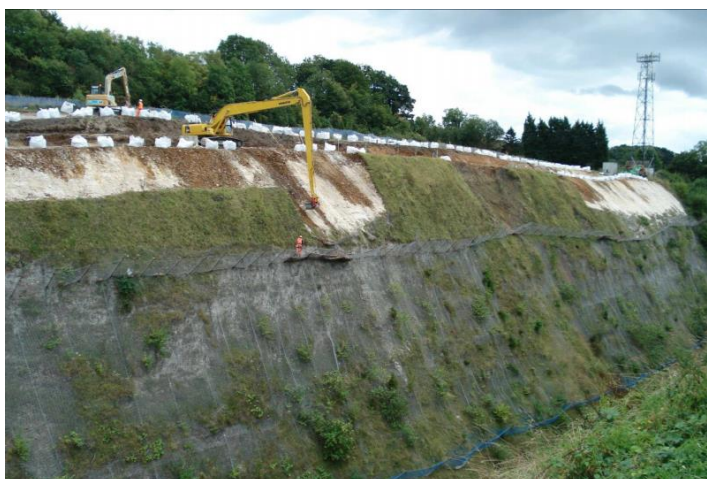
Figure 6-28 Removal of weak material at central spine of Down Redhill Cutting (O'Donovan, 2014)
