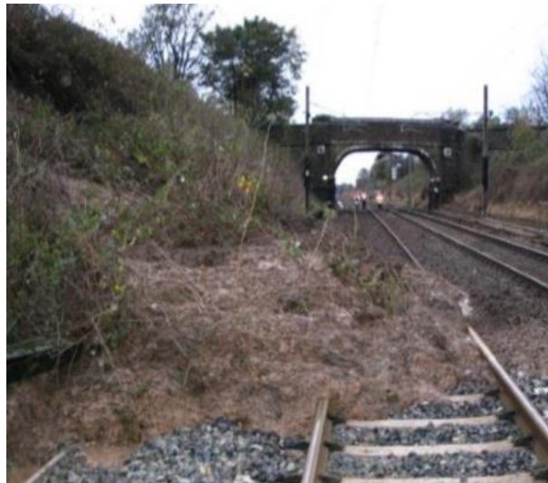
Figure 2-4 Example of earthflow failure according to NR classification system. (Network Rail, 2015a)
