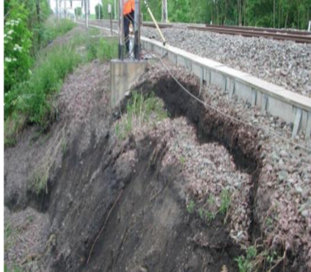
Figure 2-6 Example of rotational failure according to NR classification system (Network Rail, 2015a)
