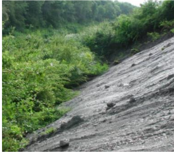
Figure 2-3 Example of translational failure according to NR classification system. (Network Rail, 2015a)
