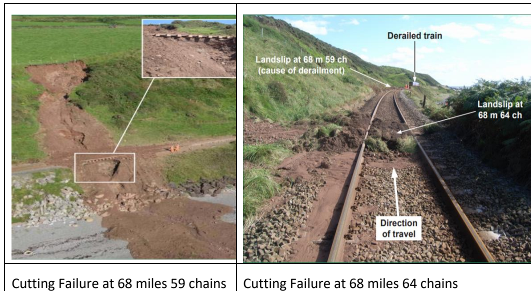
Figure 6-31 Cutting Failures at St Bees (RAIB, 2014)
