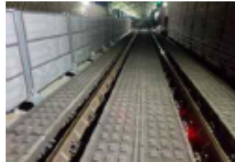
Figure 2.4. Track with absorptive blocks for the measurement [40]
