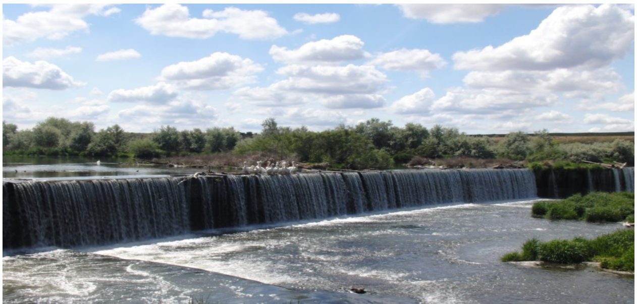
Figure 1.1 Low-head irrigation dam in the Pacific North-west of the USA. This dam provides a barrier to fish passage if no passage structures are implemented.
