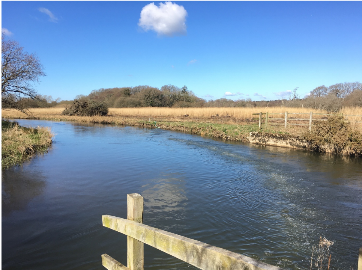
Figure 1.3 Operating bubble curtain at a diversion channel. The path of the bubbles is visible spreading from the lower right-hand corner of the photograph and spreads upstream. The purpose of the barrier is to divert fish into the bypass channel at the bottom left of the photograph.
