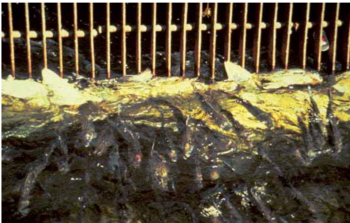
Figure 1.2 Impingement of fish at a screen. Notice the fish pressed against the screen in the upper section of the photograph and the fish swarming in the lower section. (Credit FAO)
