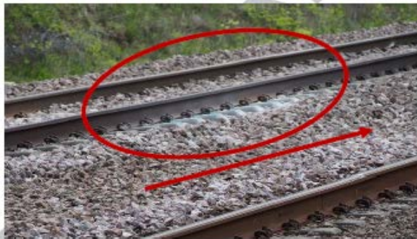
Figure 2.30: Concrete UTX site at Öbisfelde, Germany (Powrie and Le Pen, 2016)
