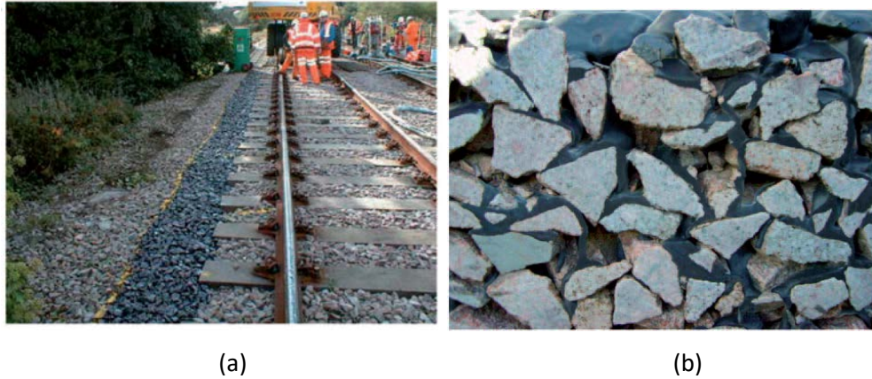
Figure 3.16: (a) Use of Polyurethane on Harford, UK, (b) cross-section (Woodward et al., 2011)
