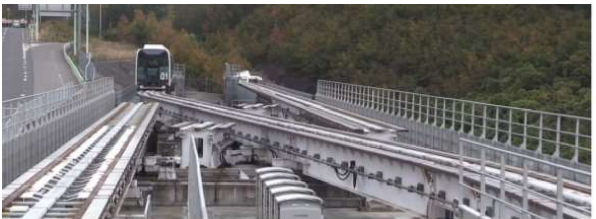
Figure 2-23: Switching system on the Linimo line in Nagoya, Japan. (Source: Thorstrand, 2020)
