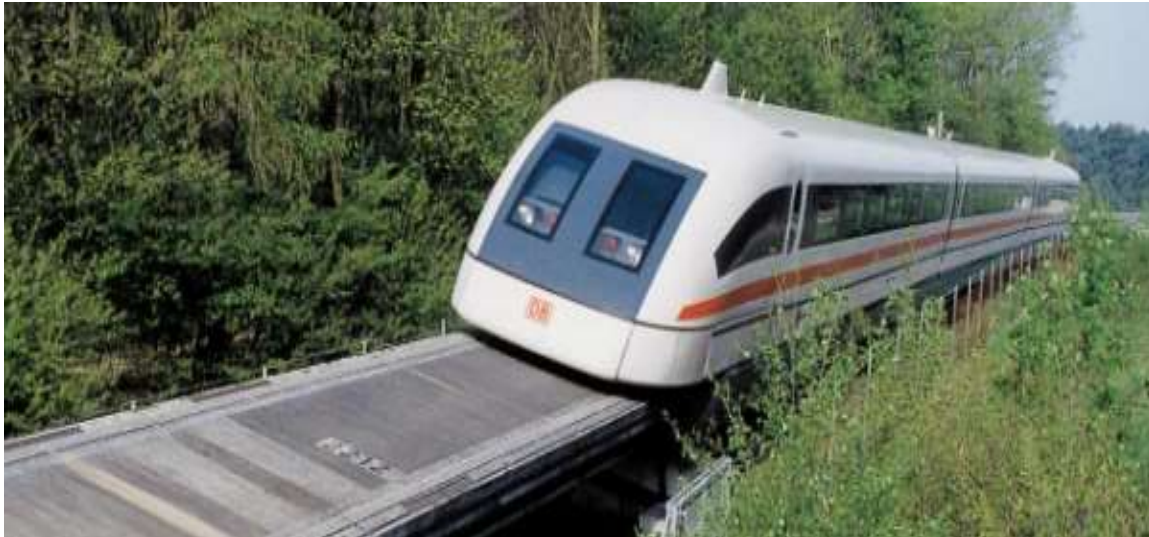
Figure 4-2: Transrapid Maglev train. (Source: Transrapid International, 2002)
