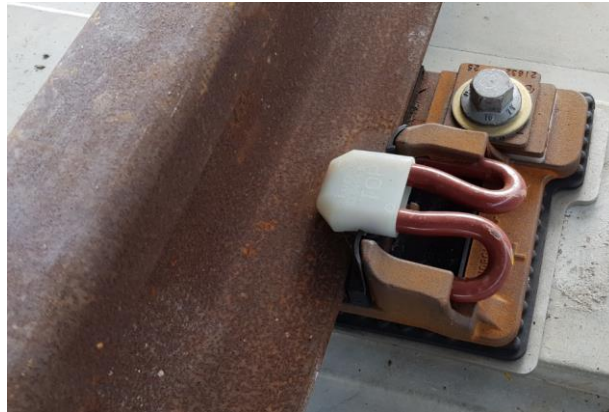
Figure 1-8 The Pandrol two-stage baseplate.
