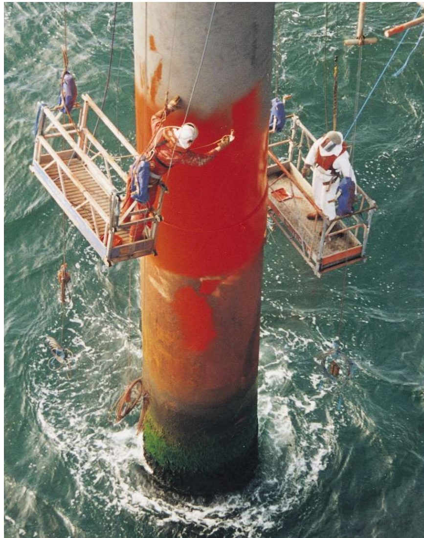
Figure 1: An example of a commercially formulated system in the field: Orange Denso Unsaturated Polyester coating protects a support pile in a marine environment. (Photo courtesy of Winn & Coales (Denso) Ltd.)
