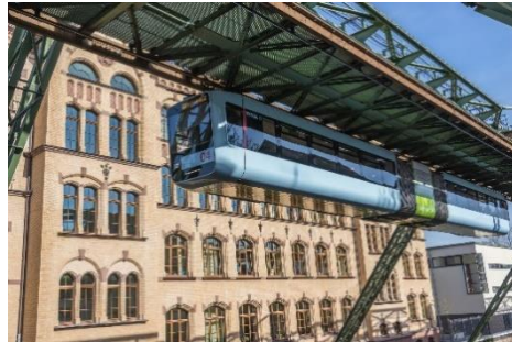
Figure 1-1 The suspension Schwebebahn Wuppertal, Germany
