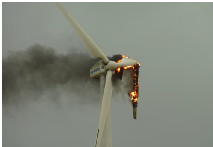
Figure 1.2 – Wind turbine damaged by a lightning strike [10].
