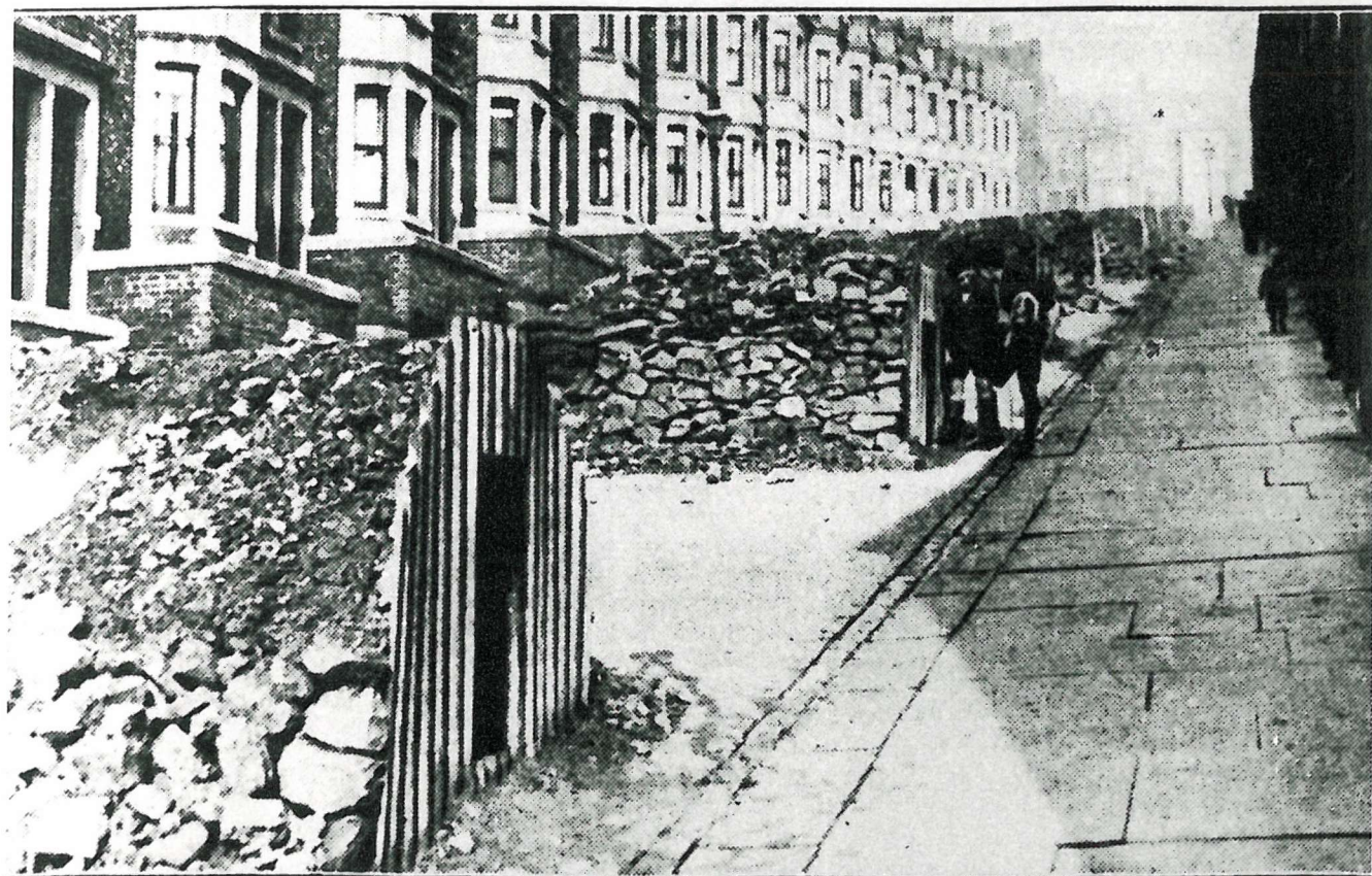
The larger type of Anderson shelter built along the whole length of a street in Newcastle-on-Tyne.
