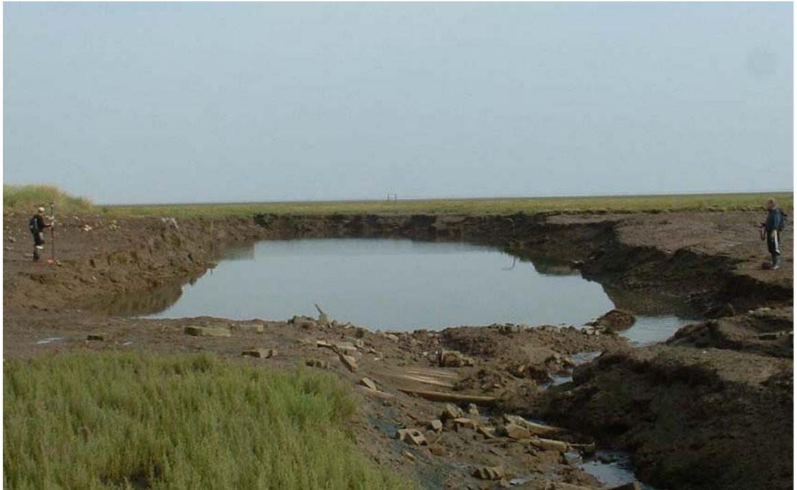
Plate 6.3: A seaward view of the channel within Breach 1, from the most recent site visit (05/09/2005). Note: the widest point of the channel was 28 m.
