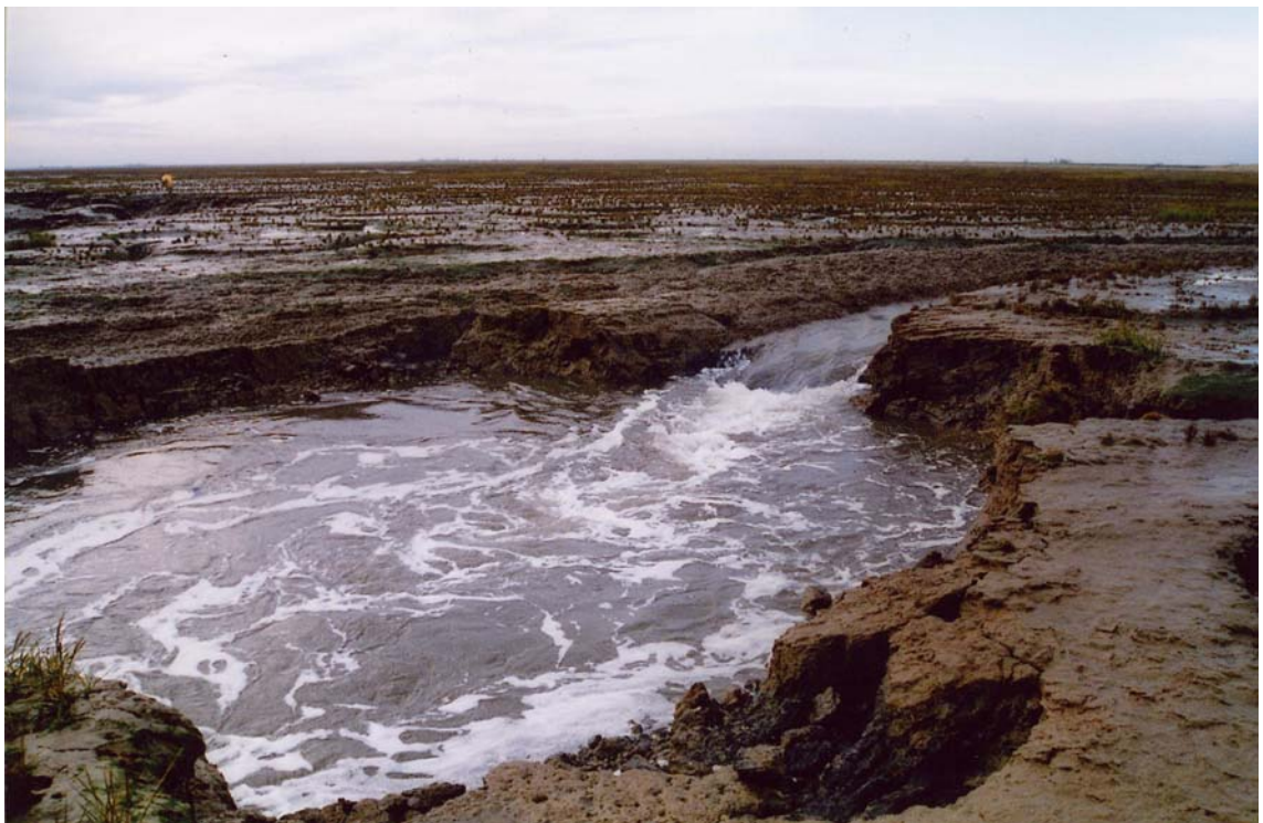
Plate 6.4: The point in the natural creek connected to the artificial channel within Breach 1, where the channel has been eroded (25/11/2003). The photograph is looking landward, the flow in the creek is from the drainage of the MR site. Note: the creek to the right is approximately 3 m in width, whilst the eroded area varies, in width, from 6 to 10 m.
