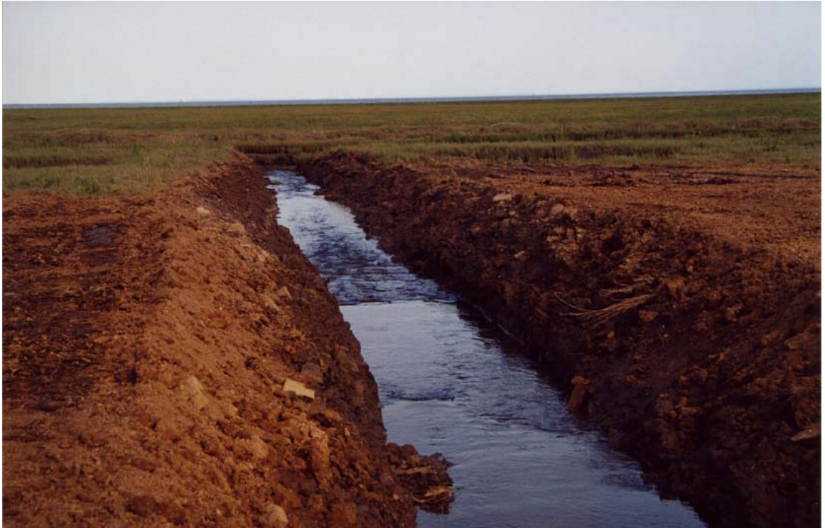
Plate 6.1: A seaward view of the channel within Breach 1, shortly after it was created (22/08/2002). Note: the width of the channel at the bed was 2 m.
