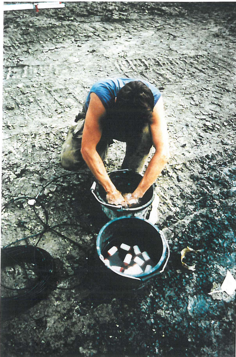
Plate 9-2. Saturated piezometer tip being assembled under water immediately prior to installation.
