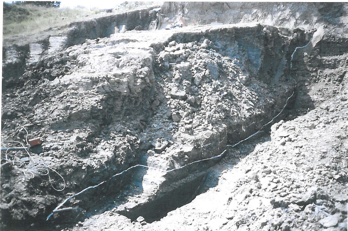
Plate 15-2. Inspection trench widened and battered back.
