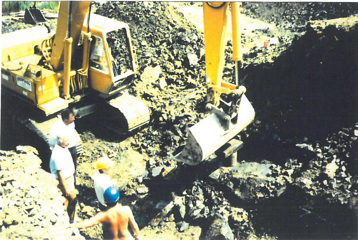
Plate 15-3. Sampling of the slip surface using 300mm dia. push samples.
