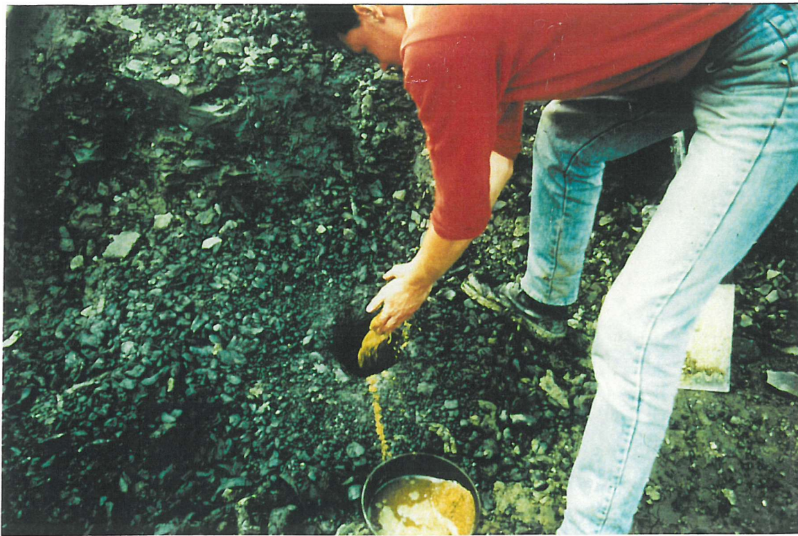
Plate 9-1. Piezometer installation. Measured quantity of saturated sand being placed in borehole to provide piezometer filter "pocket". Sand washed in with bucket of water to clean borehole walls.
