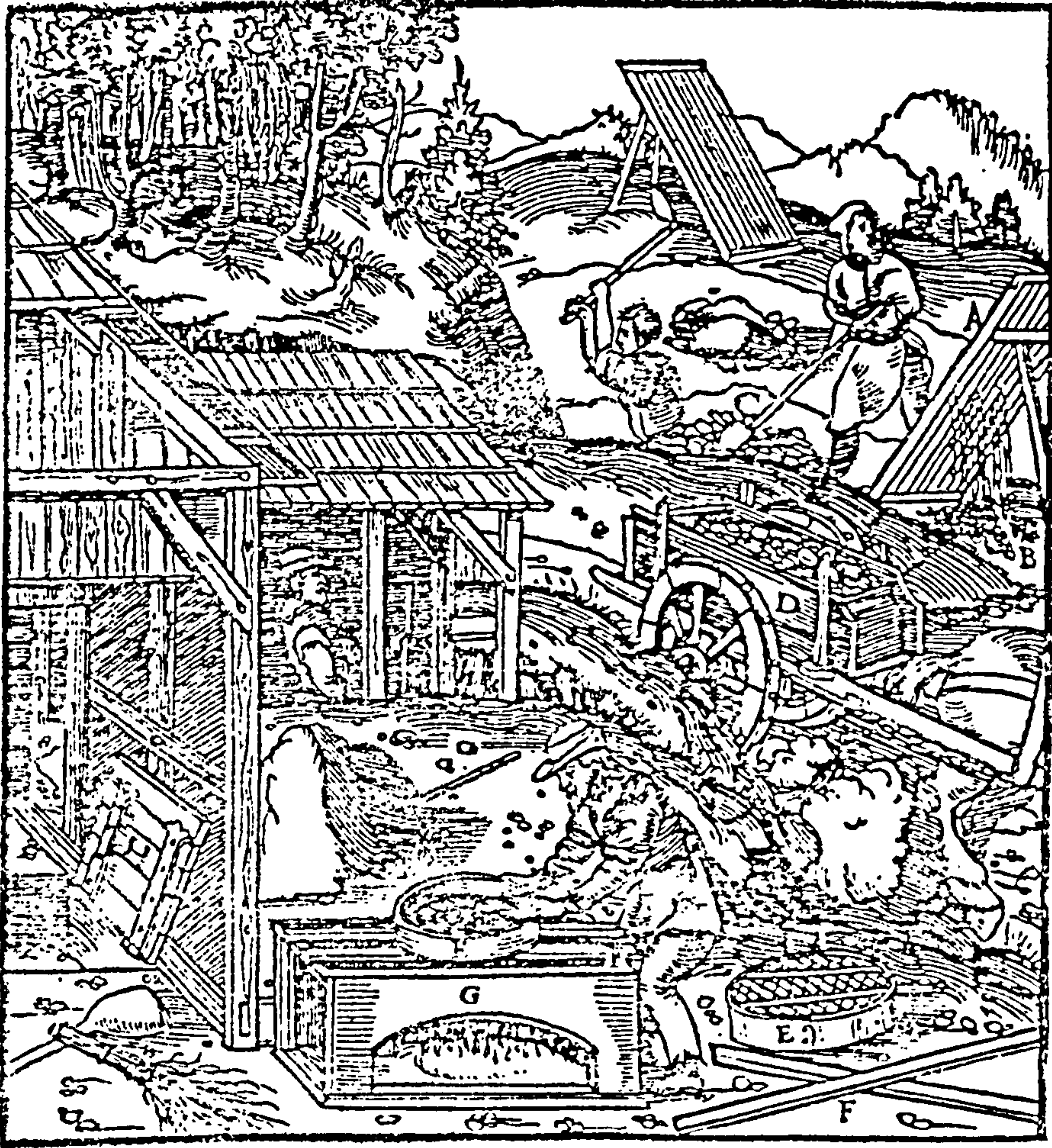
A—SCREEN. B—POLES. C—SHOVEL. D—TWO-WHEELED CART. E—HAND-SIEVE. F—NARROW BOARDS. G—BOX. H—COVERED PIT.
