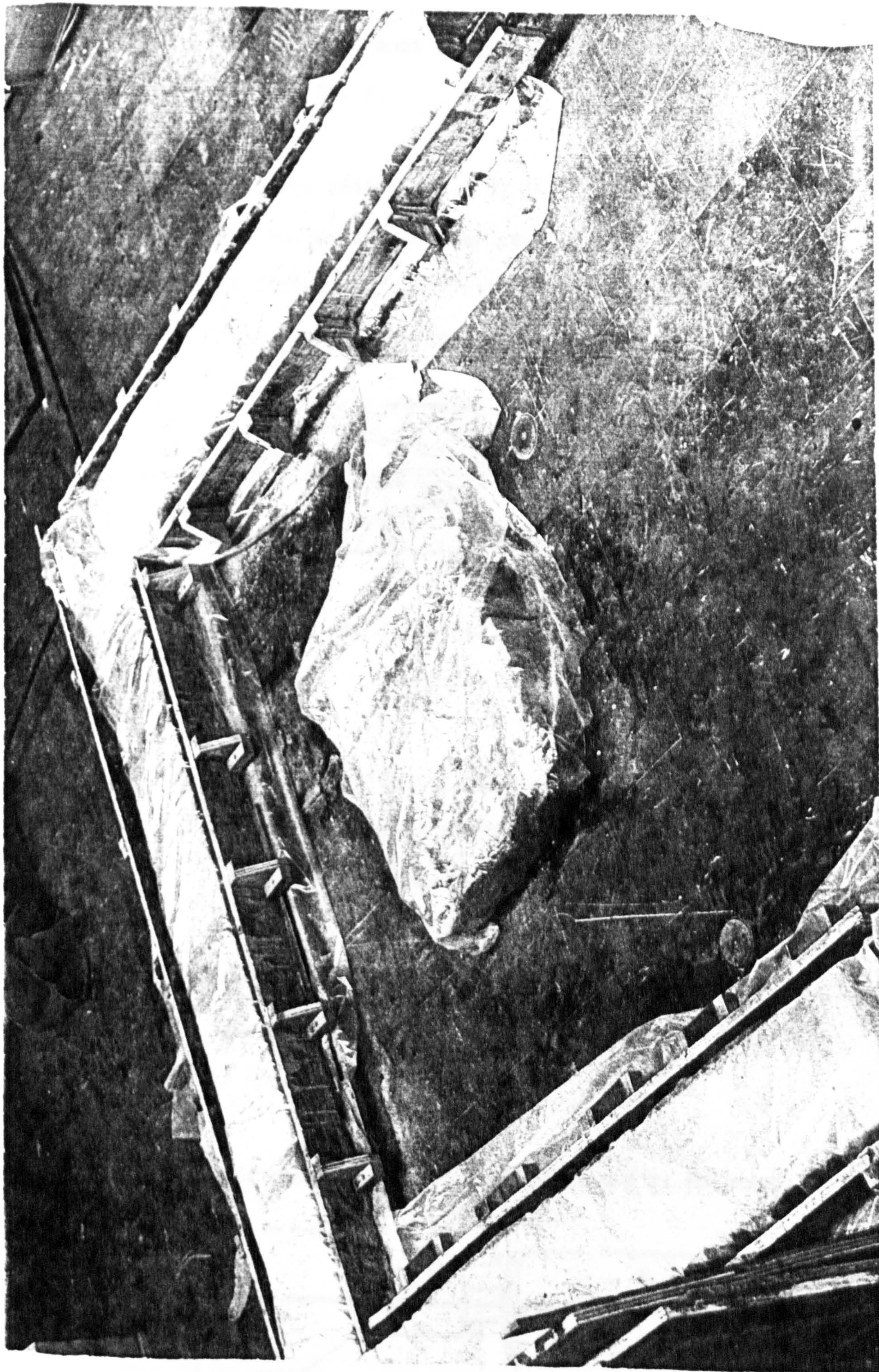
Plate No. 4 Curing the concrete
