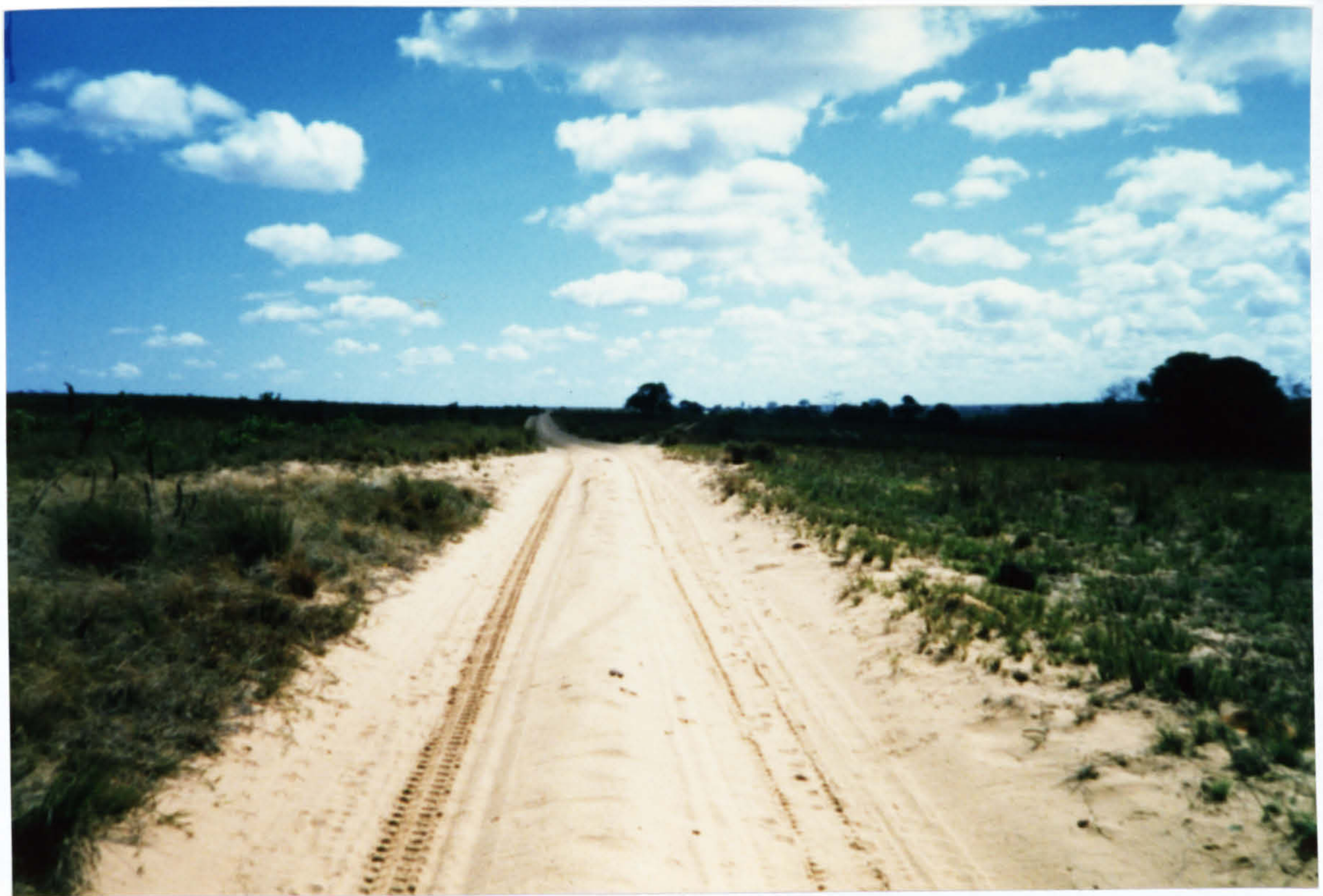
Plate 7.2 Local road to connect the communities Buena Vista and El Aceital. Guarico state
