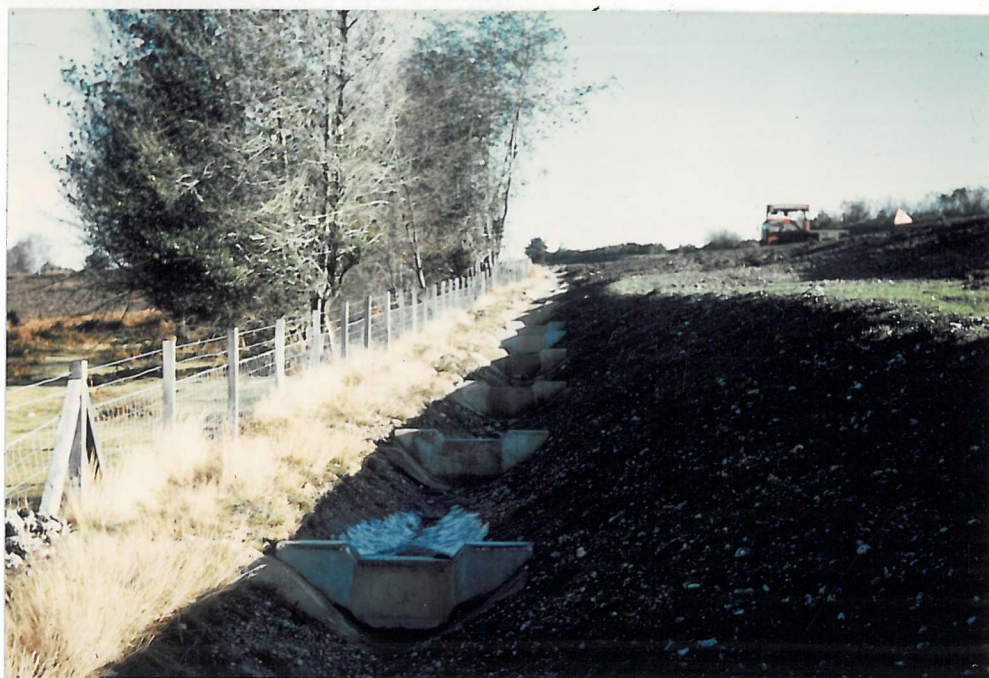
PLATE 4.4 HIGHLAND WATER: CATCH DAMS LOCATED WITHIN CATCH DRAINS IN AN ATTEMPT TO ARREST EROSION (SITE 7).
