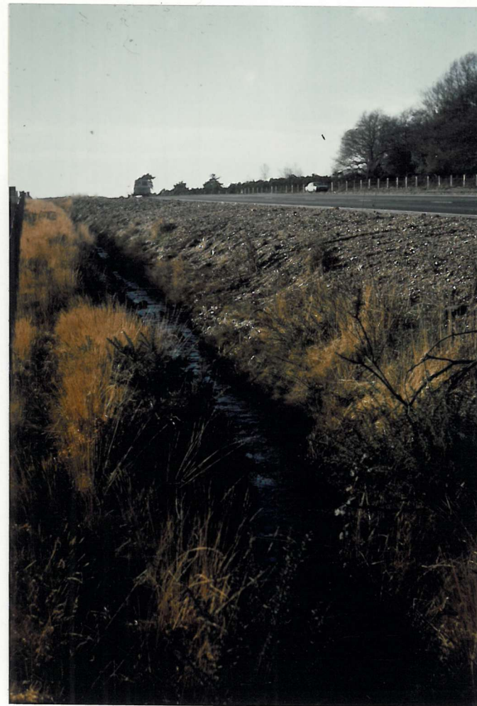
PLATE 4.3 HIGHLAND WATER: MAJOR ROAD CATCH DRAIN OF PERENNIAL/INTERMITTENT REGIME (SITE 11).
