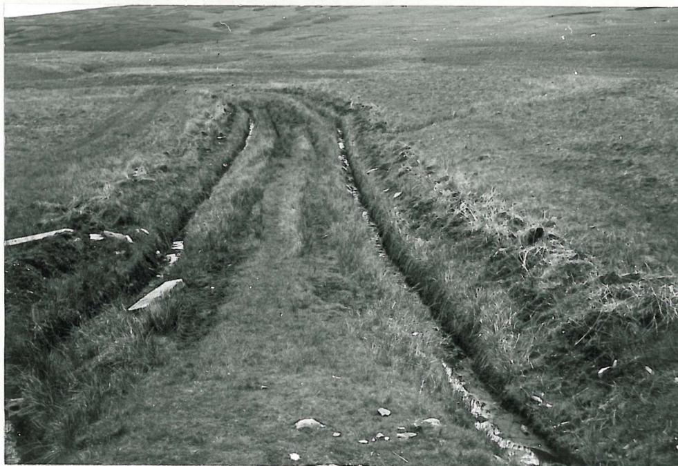
PLATE 5.13 MANOR WATER: CATCH DRAINS ALONGSIDE A TRACK HAVE RESULTED IN FLUSH METAMORPHOSIS (SITE 17) .
