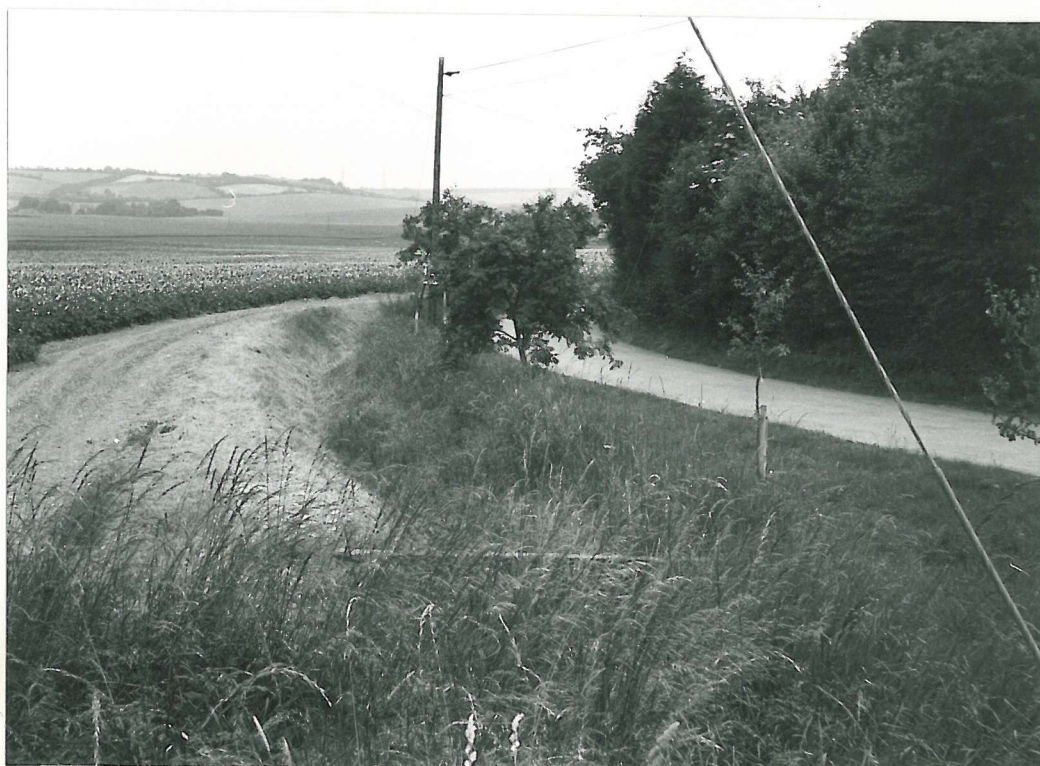
PLATE 5.21 EAST STOUR: A DUAL PURPOSE FIELD BOUNDARY AND CATCH DRAIN OF INTERMITTENT/EPHEMERAL REGIME (SITE 23).
