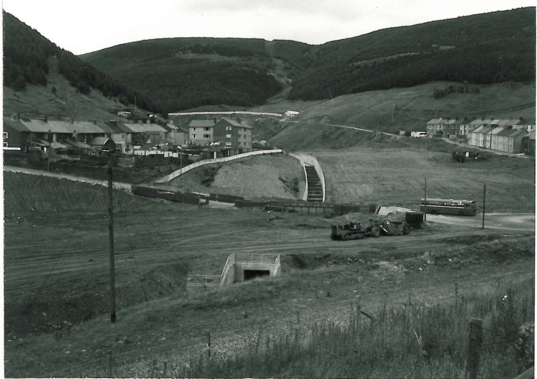
PLATE 5.24 AVAN: CONCRETE CHANNELS AND STEEL WATERFALLS GUIDE THE RE-ALIGNED CHANNEL (SITE 37) THROUGH A RECLAIMED TIP AREA.
