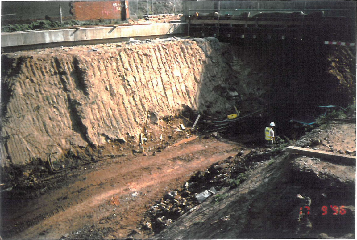
Figure 3.9. Bulk excavation, leaving behind temporary earth berms
