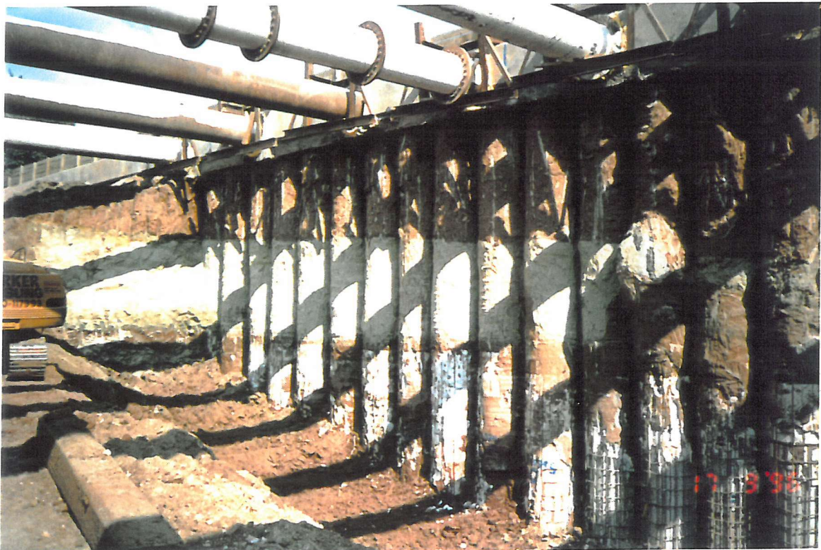
Figure 3.10. Temporary props pre-loaded and earth berms excavated
