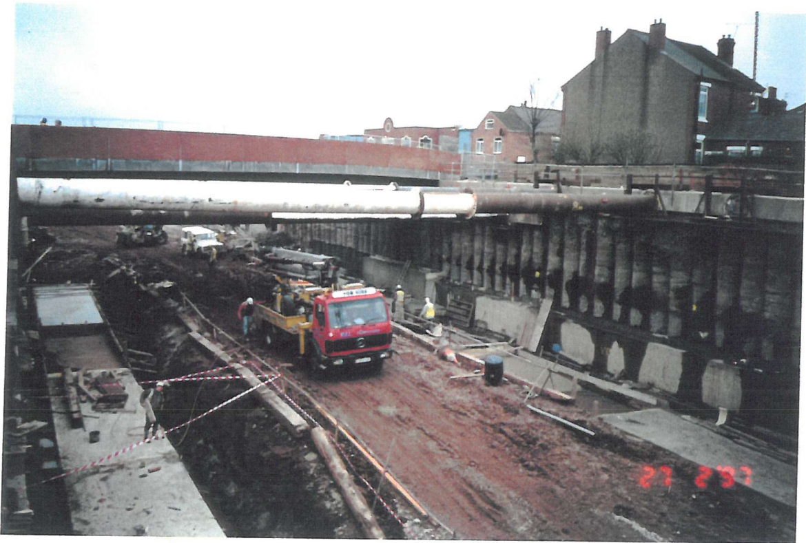
Figure 3.11. Stabilising base constructed and temporary props being removed
