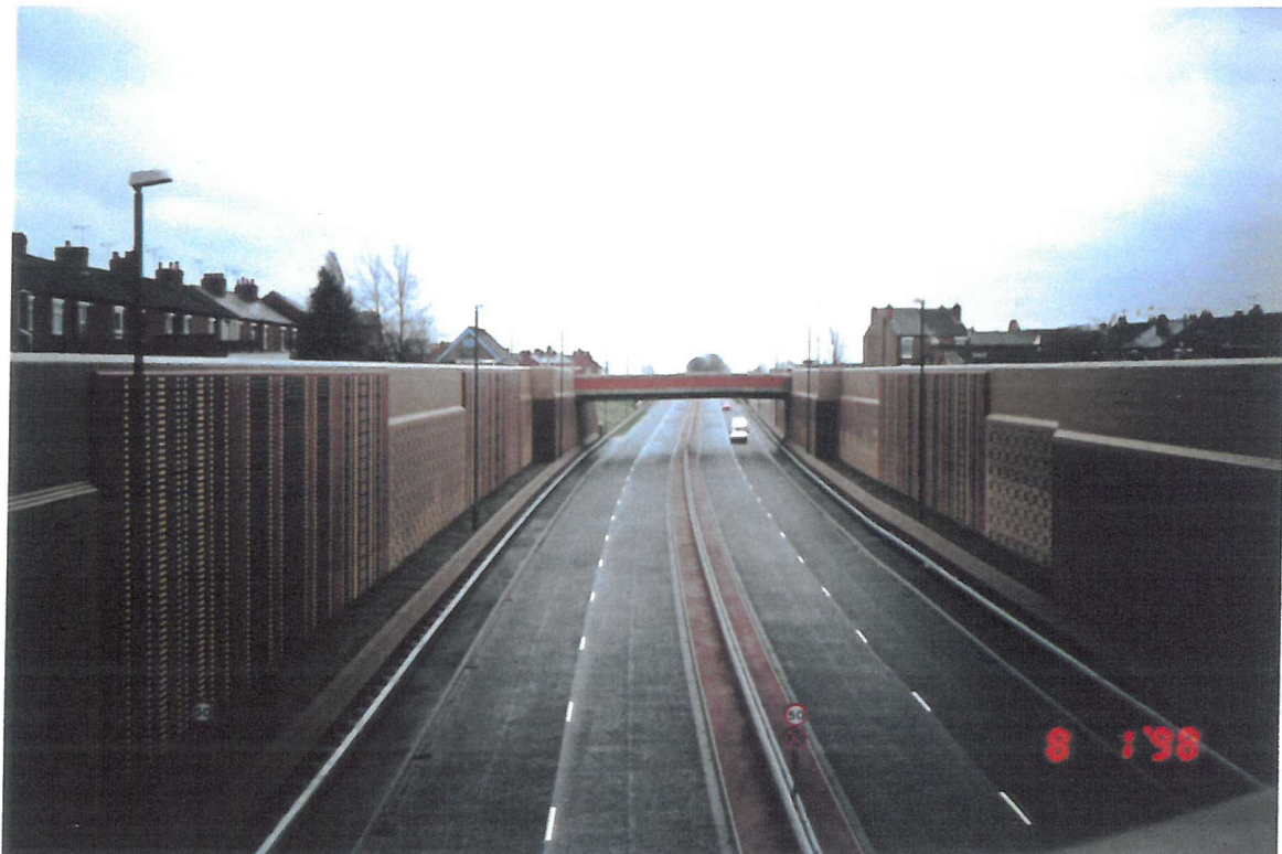
Figure 3.12. Road open to traffic
