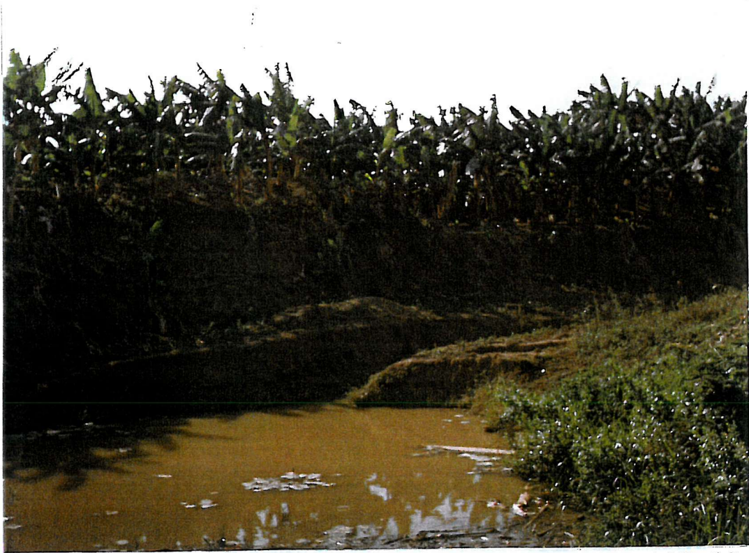
Plate 6.1: Drainage channel erosion scars following a period of heavy rainfall activity
