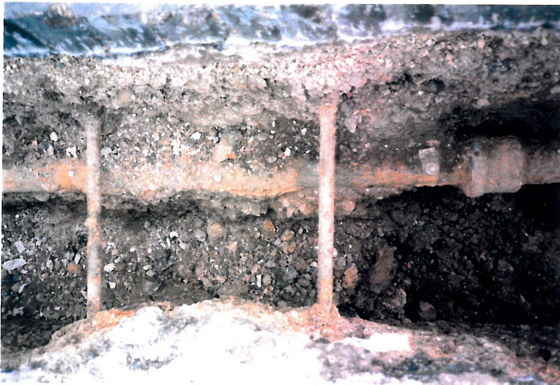
Figure 5 Small diameter pipes crossing path of 3" pipe; also Joint C and capped ferrules.
