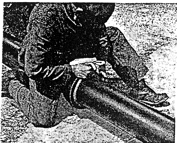
Fixing the asbestos rope runner
