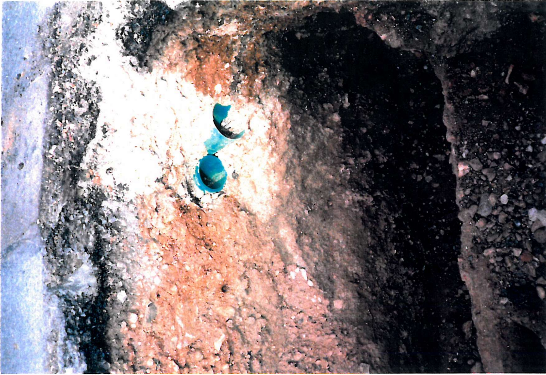
Figure 6 Cable conduits with backfill (north end of trench)
