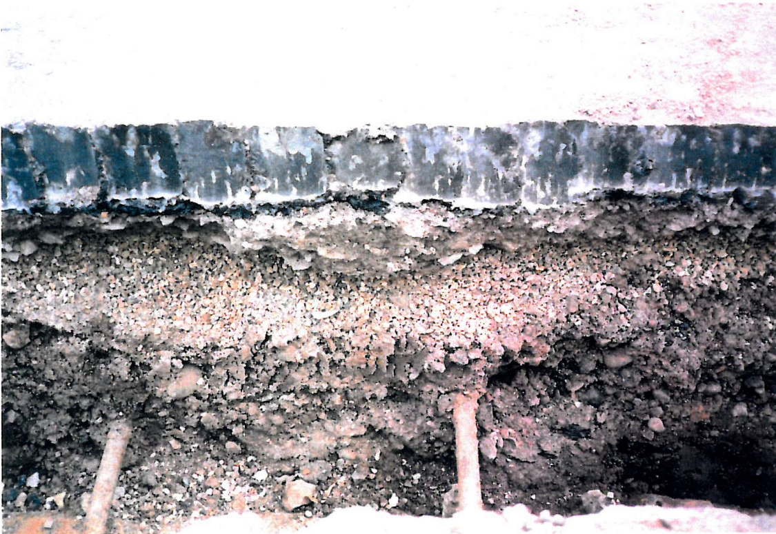
Figure 7 Patch repair, showing pea gravel
