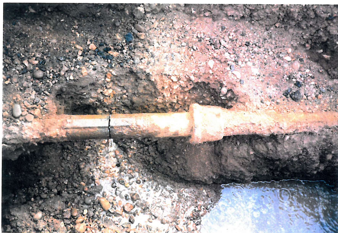
Figure 15 Wetted trench conditions, after cutting pipe
