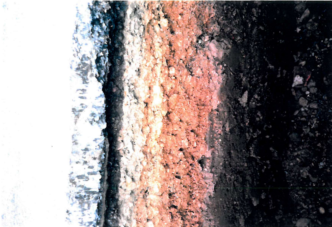
Figure 4 Side wall of trench, showing asphalt, road sub-base layer and pipe backfill
