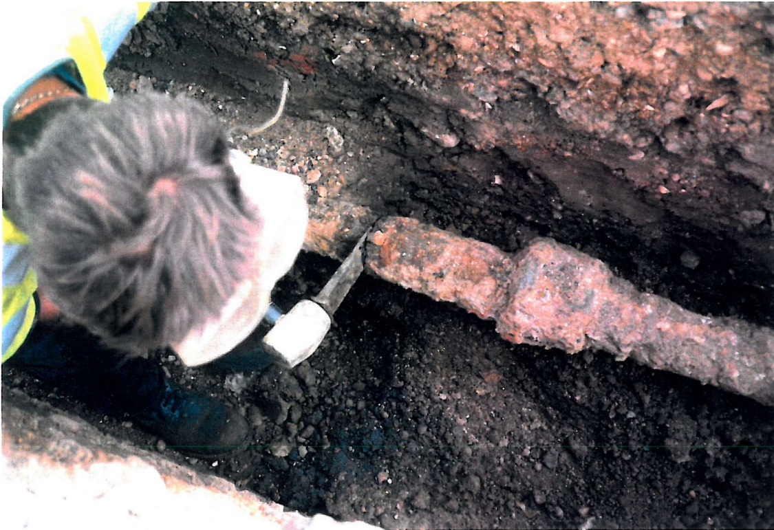
Figure 8 Use of wedge in removal of pipe segments
