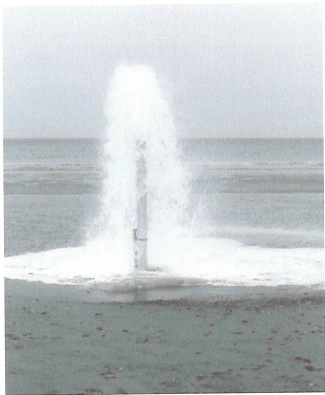
Figure 2.5: Drainage system outfall, Holme Beach, Norfolk
