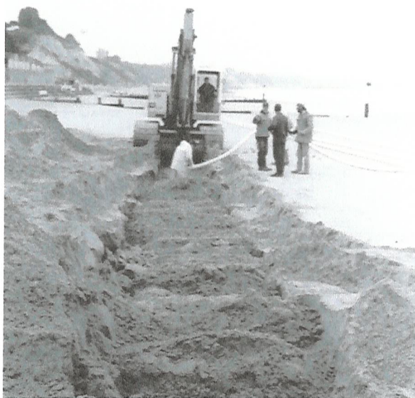
Figure 3.17: Installation of beach drainage pipe
