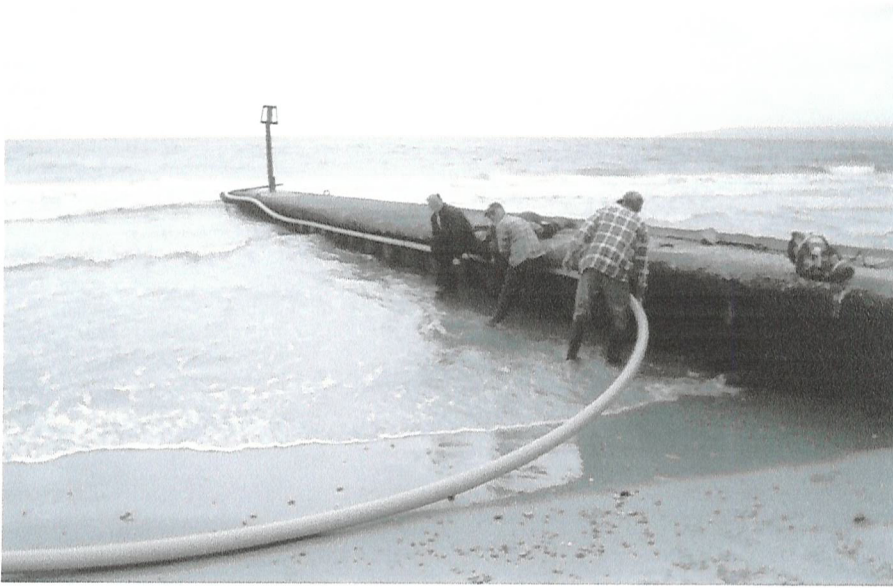
Figure 3.19: Sump outlet being fixed to the concrete groyne
