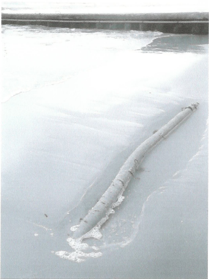
Figure 3.31: Uncovered beach drain 6/9/98
