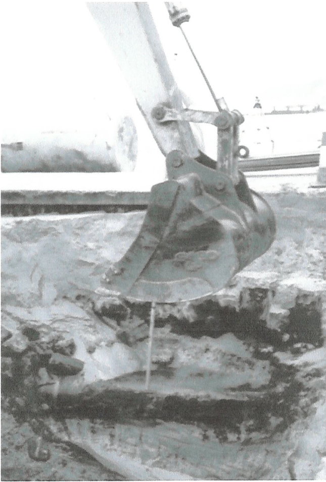
Figure 3.3 Soil profile revealed during sump excavation
