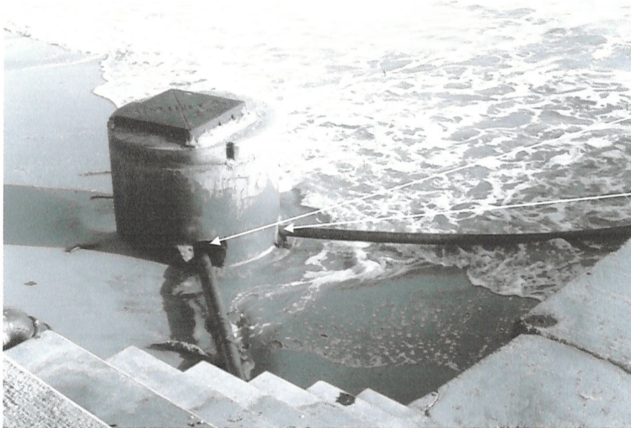
Figure 3.34: Damage to concrete seal around power inlet
