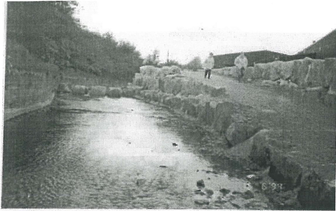
Figure 3-1: The Newly Constructed Gravel Trap on the Shelf Brook in 1994
