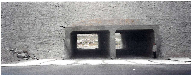
Figure 7.4 Large box culverts along the railway line.
