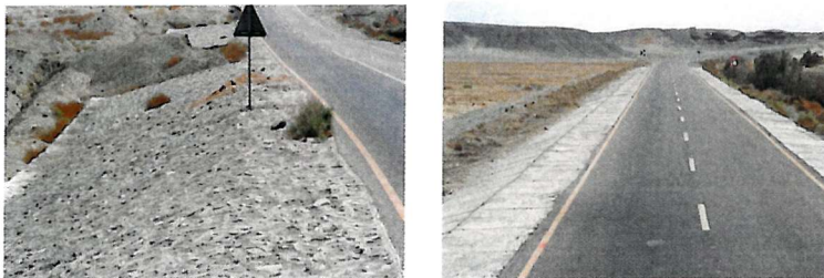
Figure 7.3 Bridgeless crossing along the Red Sea coastal road.
