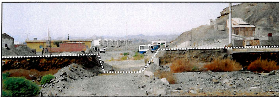
Figure 7.6 Part of the pedestrian walkway damaged by a flood in 1996 due to the small size of the culvert that constructed under it. The line annotated runs along the length of the walkway and shows the general vertical profile after the flood damage in the bottom photo.
