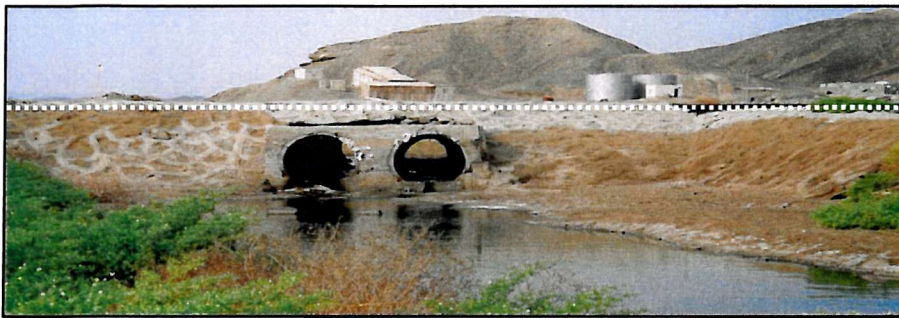
Figure 7.5 Small culvert for passing the flood water under the pedestrian road.
