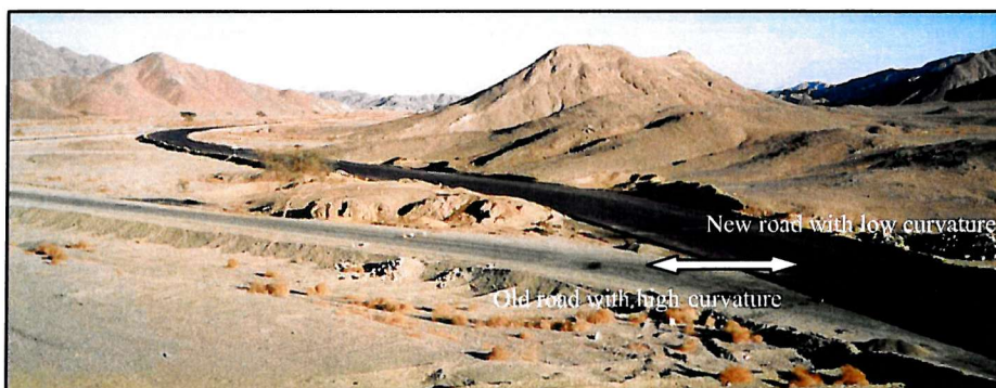
Figure 7.7 Oblique view of the Idfu-Marsa Alam road crossing through the Wadi El Alam. Note the low culvert of the new Idfu-Marsa Alam road that suits fast modern traffic.
