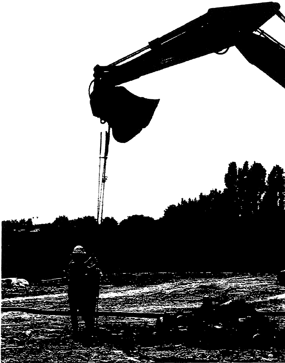
Figure 3.8: Reinforcement lowered into the fluid concrete by hand, helped by the back actor when necessary
