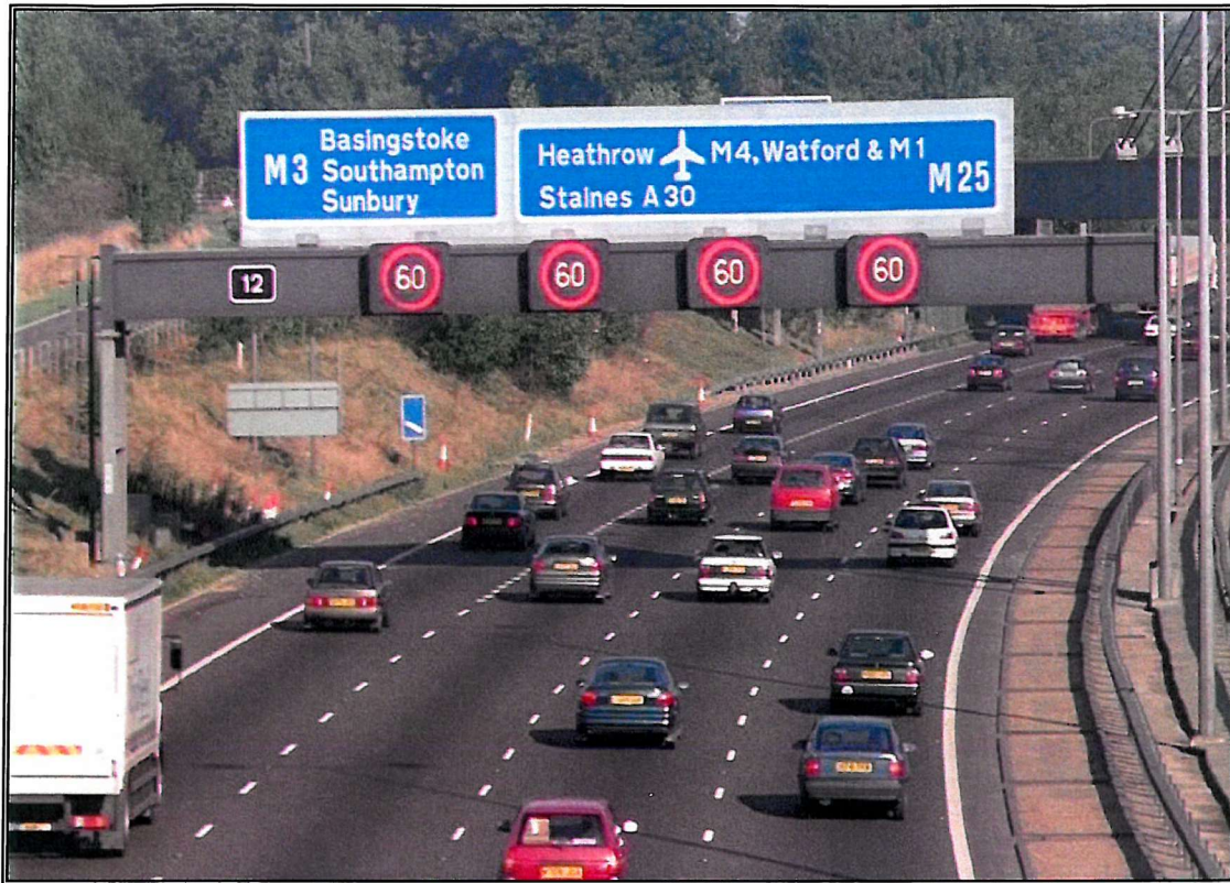
Figure 2 – Variable Speed Limits in operation as part of Controlled Motorways on the M25 London Orbital between J10 and J16
