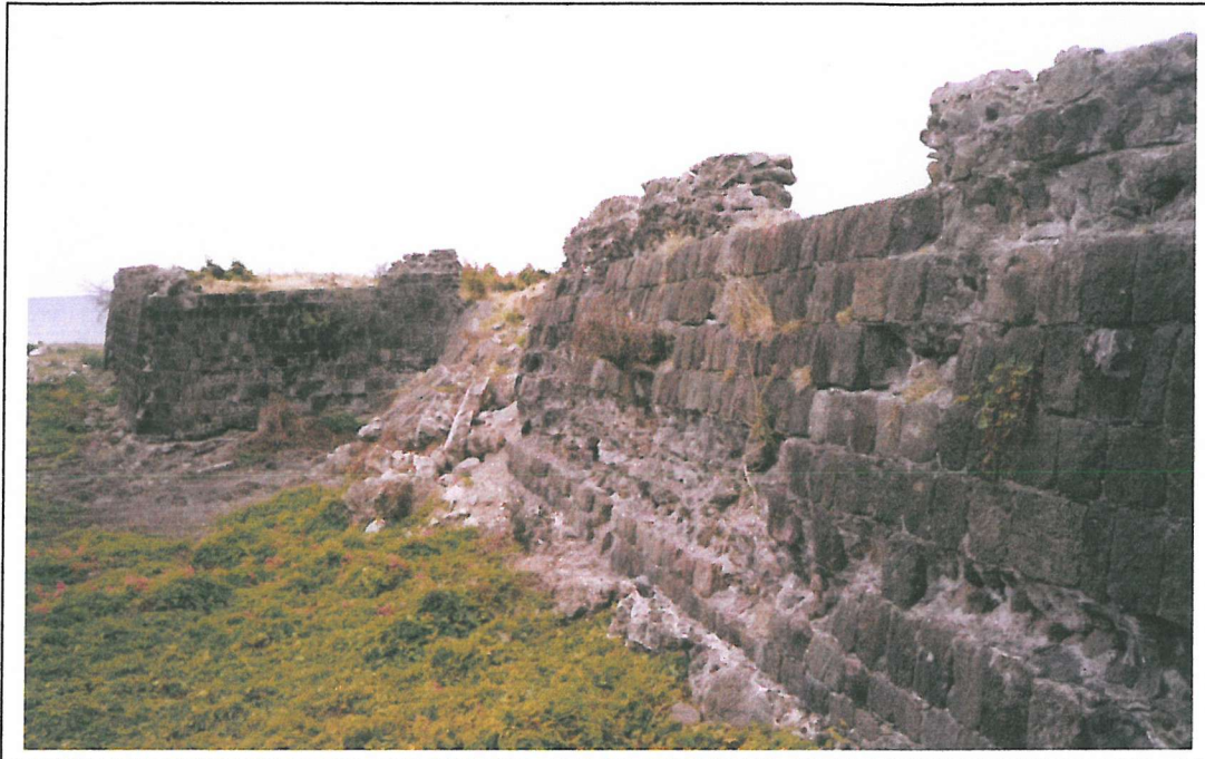
Figure C9d) Southern wall and south-east demi-bastion of Charles Fort with wall collapse caused by robbing
