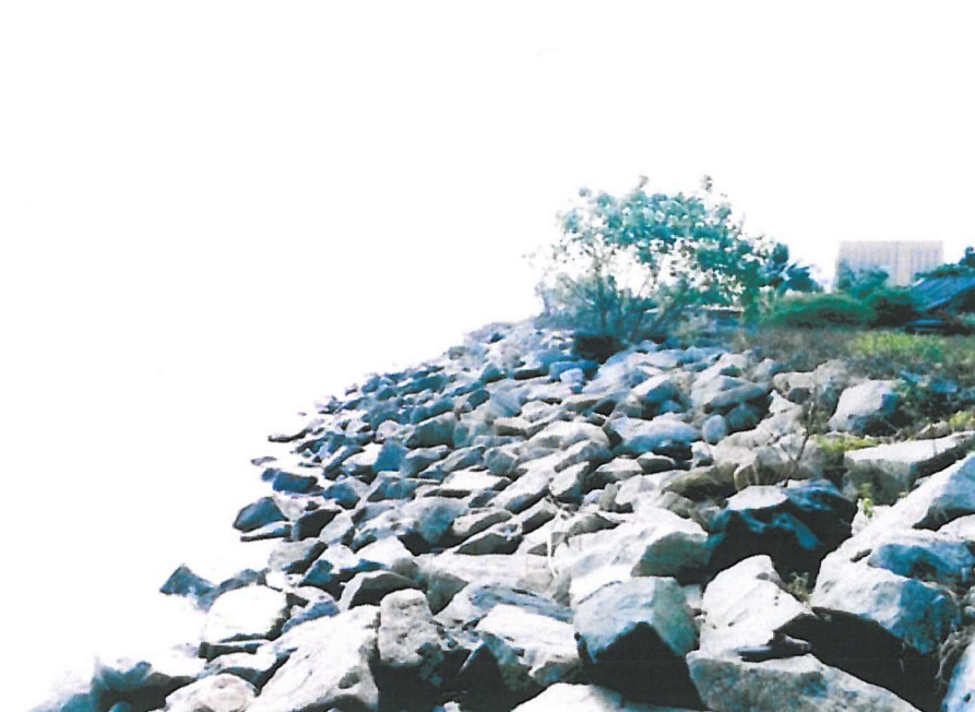
Figure 2.4: Rock sea walls were build to address coastal erosion in Kuala Terenganu.
