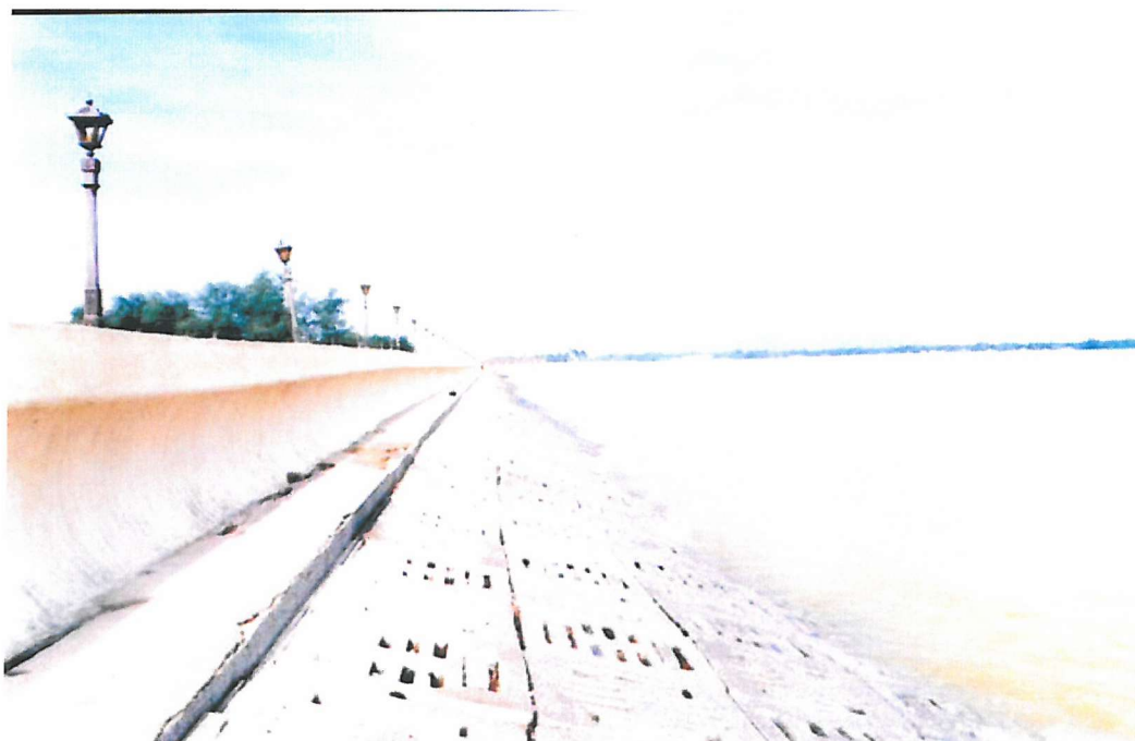
Figure 2.3: Among measures to address coastal erosion are to build a concrete seawall (Kuala Terengganu).
