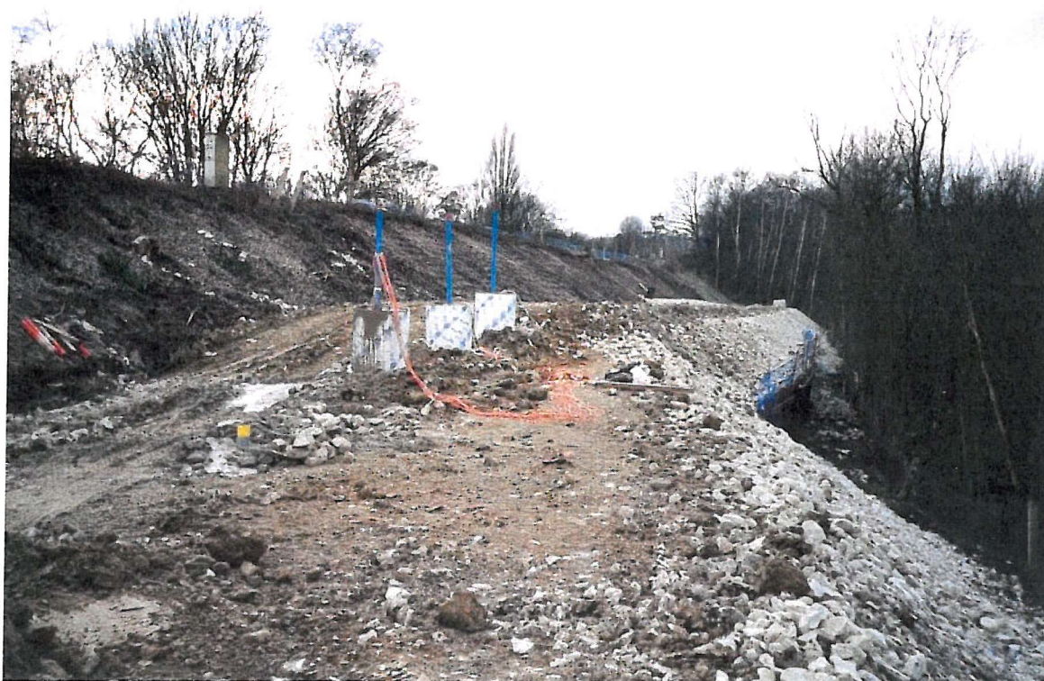
Figure 3.3. The instrumented section of the embankment at Hildenborough shortly after pile construction.
