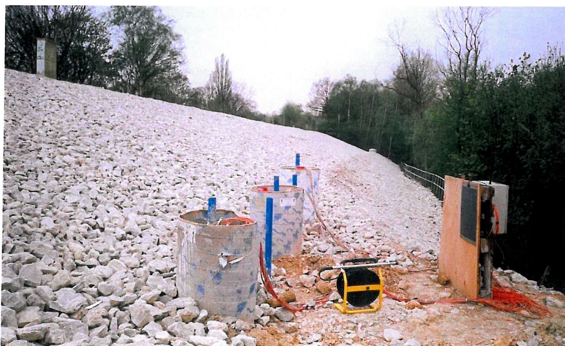
Figure 3.4. The instrumented section of the embankment at Hildenborough after the berm had been re-graded to create a two stage slope
