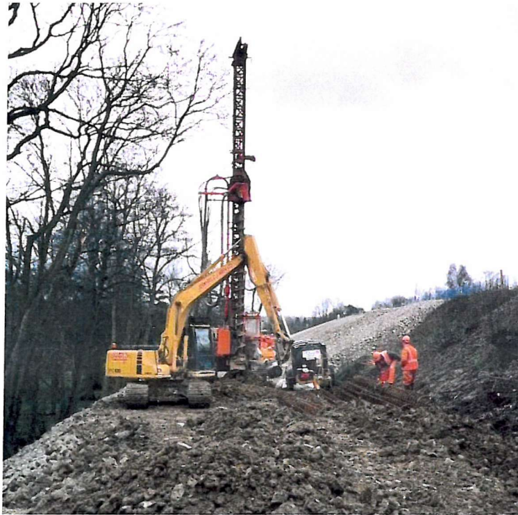
Figure 2.6. Rockfill berm constructed at the toe of a railway embankment at Hildenborough, Kent, to provide a platform from which to operate piling plant.
