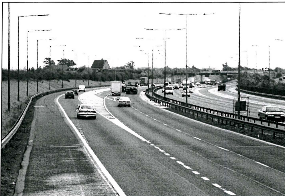
Figure 3.5: The start of the Ghost Island layout at the M6 junction 4a
